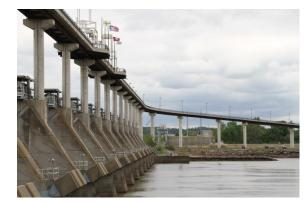
A There are 18 locks and dams - 13 in Arkansas and 5 in Oklahoma; each lock chamber is 110' wide x 600' long and can handle an 8-barge tow.
