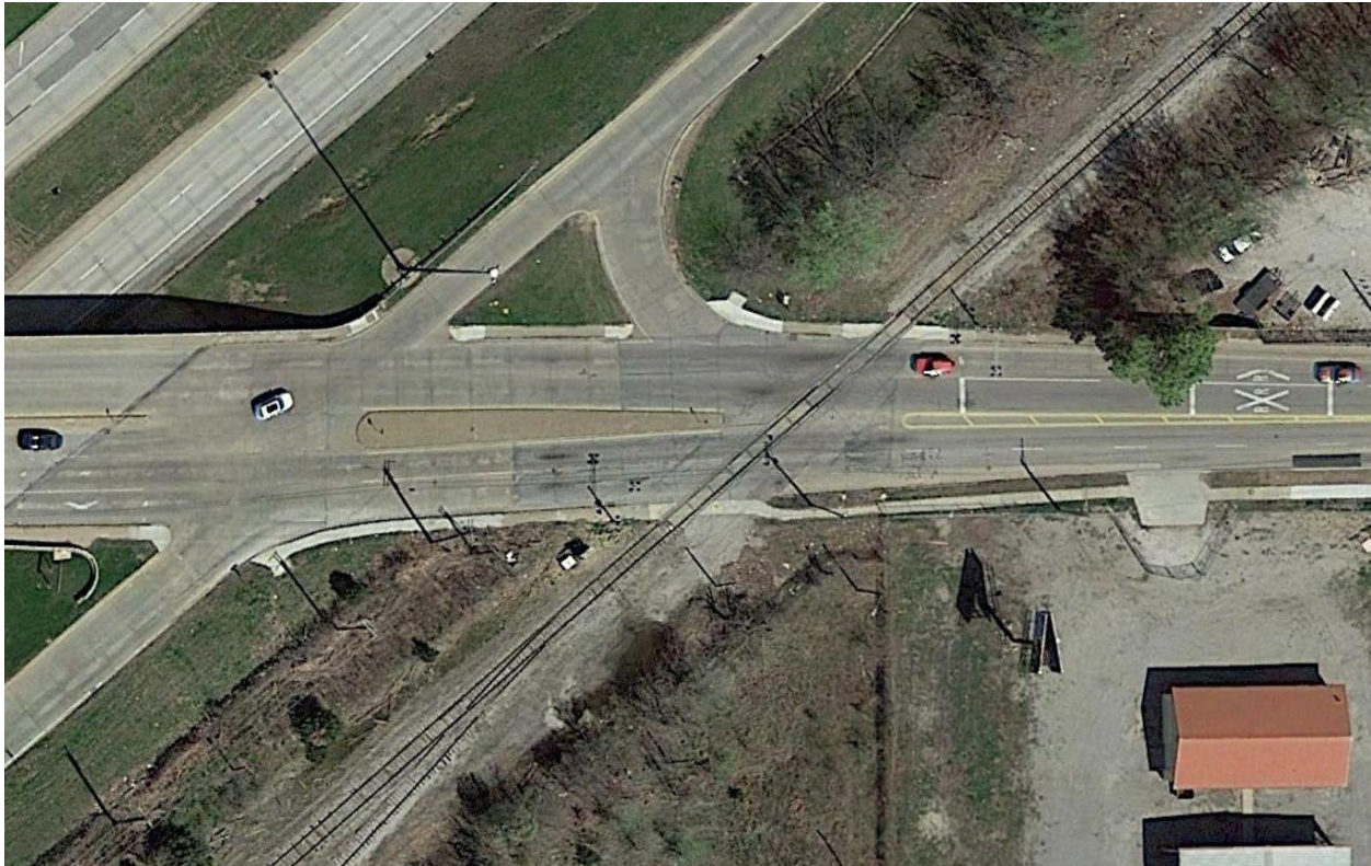
Figure 5: Pine Street on the SKO in Tulsa (DOT#-008588A)
