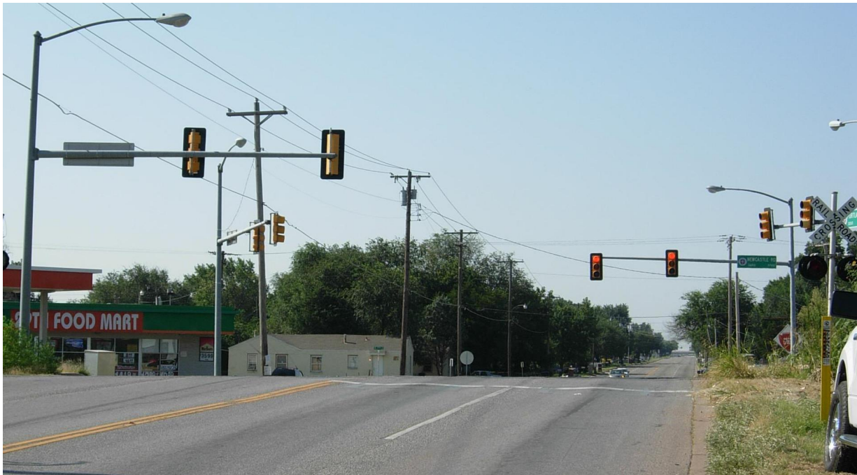
Figure 8: Portland Avenue on the SLWC in Oklahoma City (DOT#-669047W)
