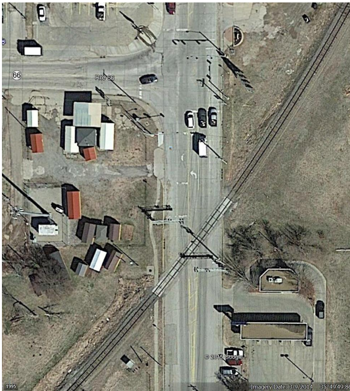
Figure 7: Main Street (SH-16) on the SLWC in Bristow (DOT# 668769A)
