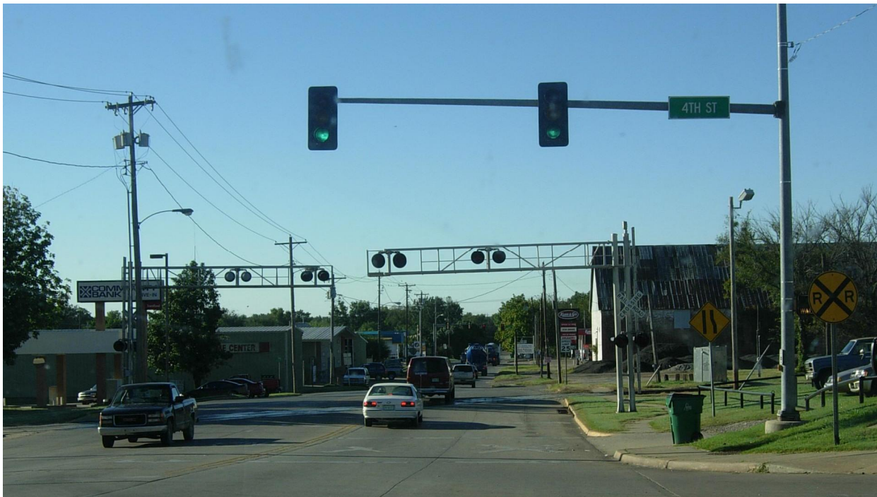
Figure 5: Main Street on the SLWC in Bristow (DOT# 668769A)
