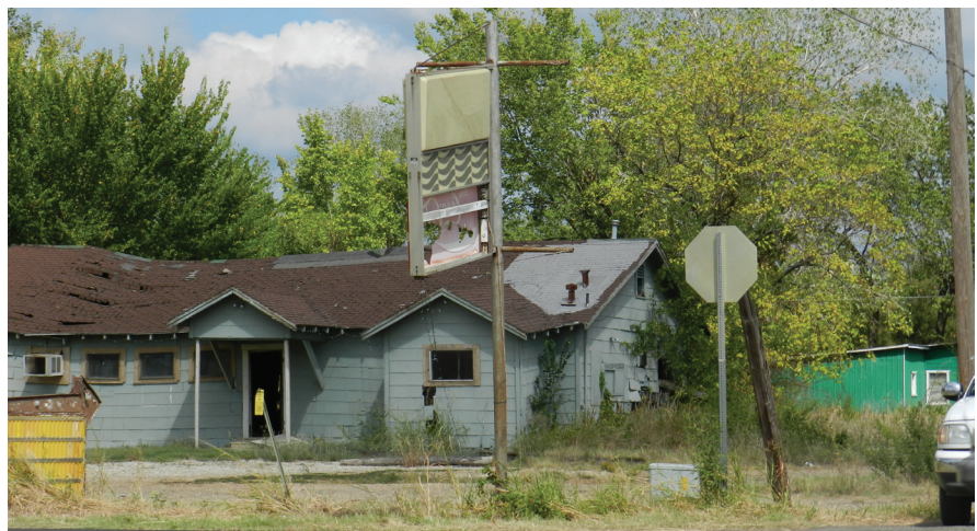
Exhibit 14: Dilapidated Structure on US 70
