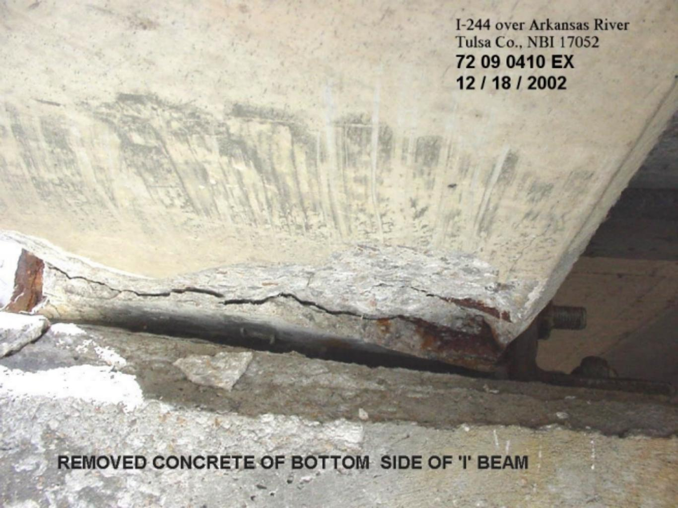
**REMOVED CONCRETE OF BOTTOM SIDE OF 'I' BEAM**
