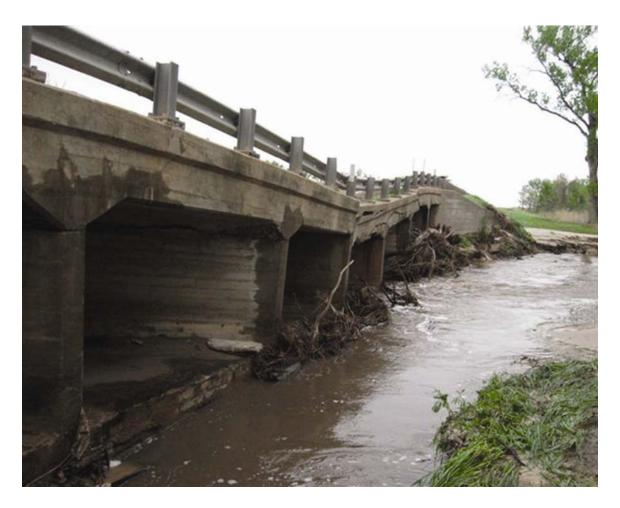
At the Oklahoma Transportation Commission's May 19 meeting, commissioners approved an emergency \$800,000 contract for a temporary structure to replace this bridge on SH-8 near Aline in Alfalfa County. The original concrete box structure, built in 1951, was heavily damaged by intense rains on April 27. It carried about 900 vehicles daily.
