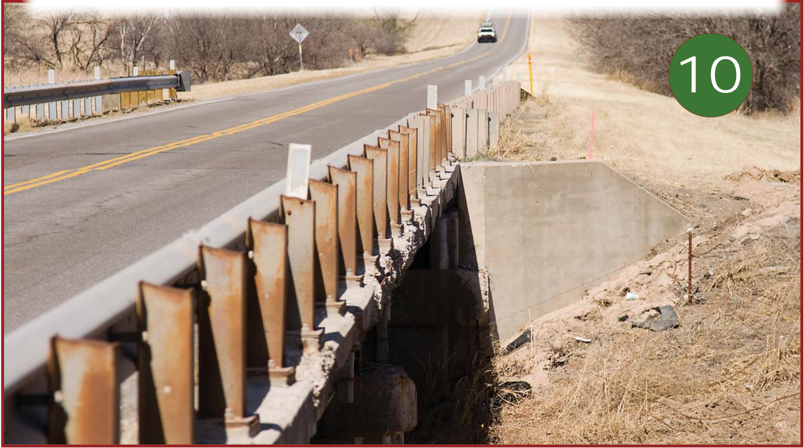
Ellis County: US-283 over Twenty-five Mile Creek near Shattuck
