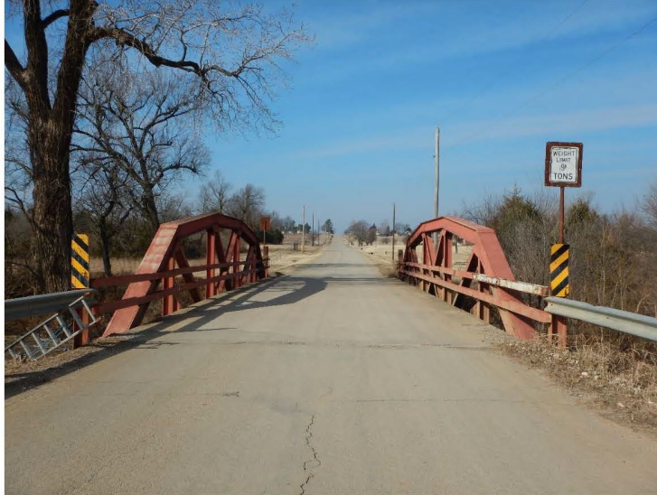
Photo 1-Bridge From East Approach With 9T Posting Sign
