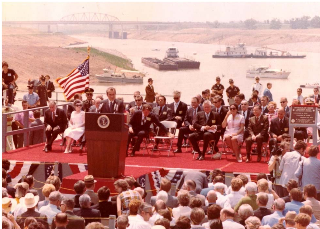
Photo 2 – In 1971, President Richard Nixon attended the inaugural opening of the McClellan-Kerr Arkansas River Navigation System in Catoosa. One of the nation’s largest, most-inland seaports, the Port of Catoosa has more than two million tons of cargo passing through it each year.
