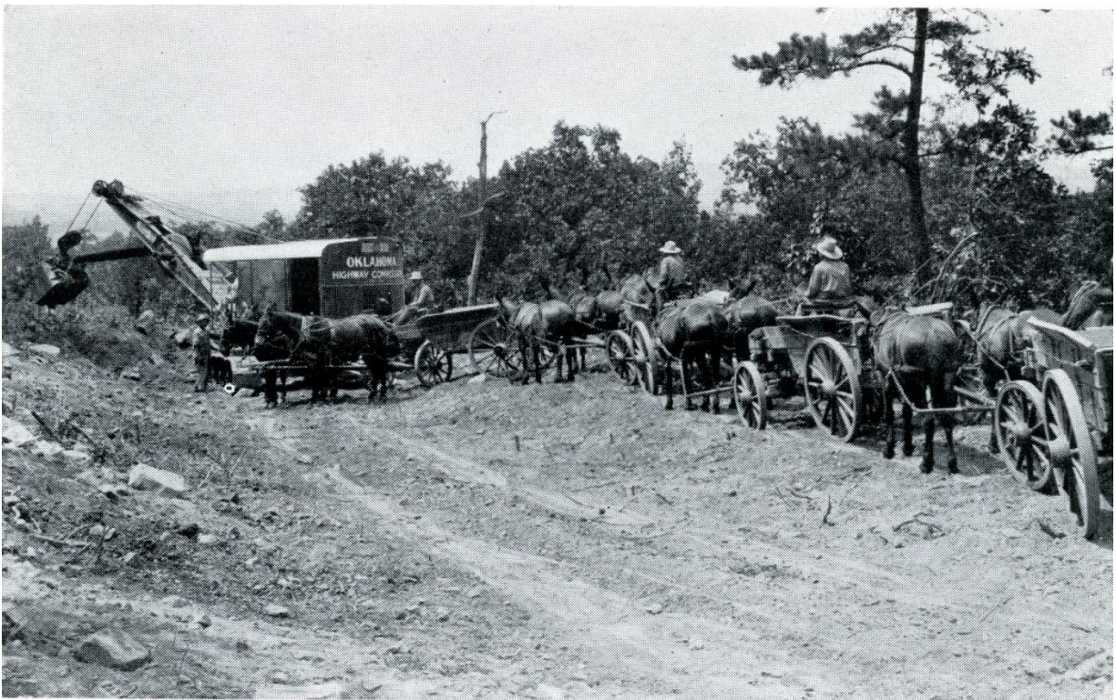
Convict labor was a cheap and available source in the early days of Oklahoma's road construction. In this photo, convicts are constructing SH-43 in Latimer County. There were no guards; the threat of going back behind "the walls" was enough to keep workers on the straight and narrow.
