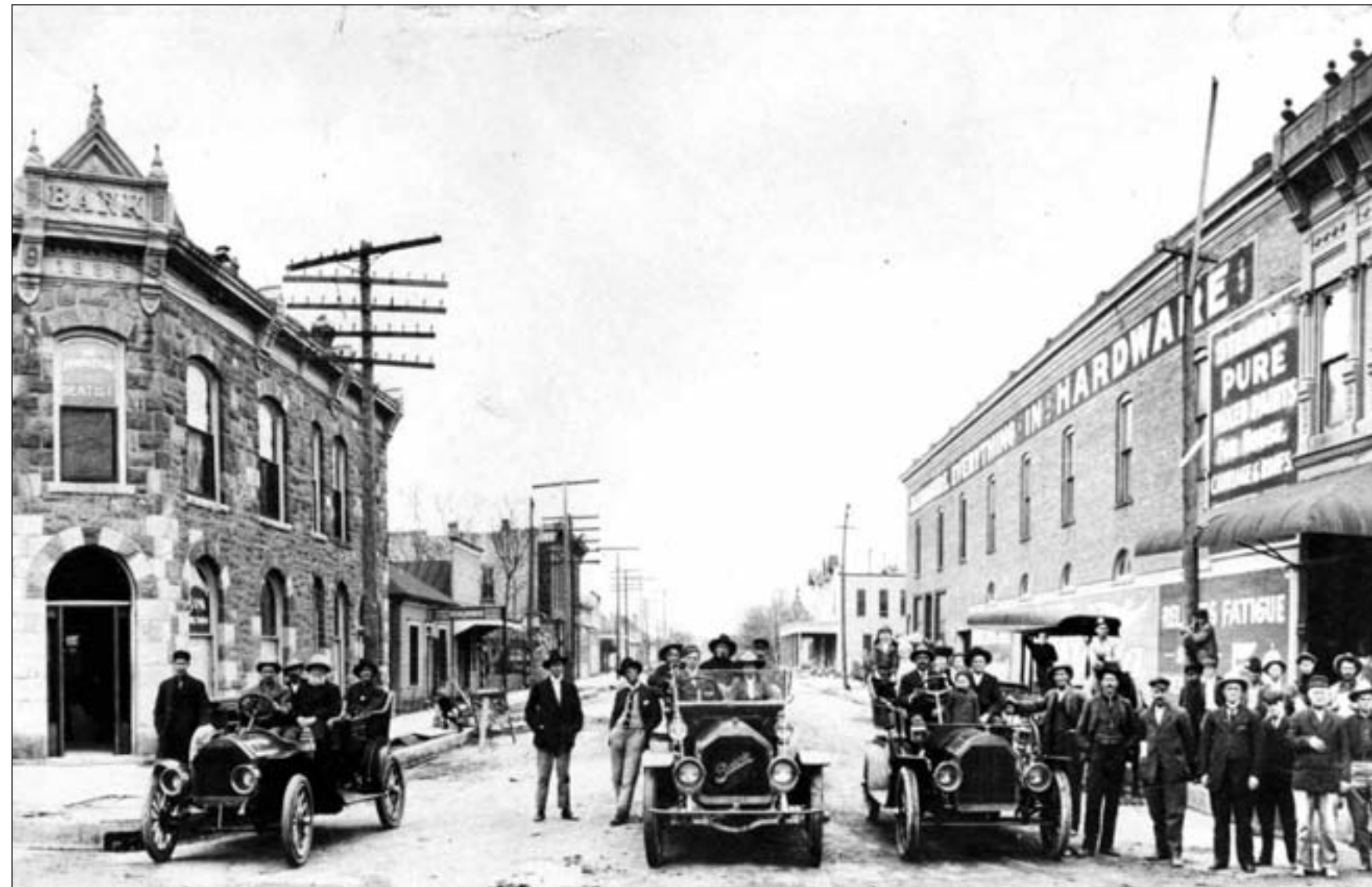
Beaver, Oklahoma in 1910 shows the presence of automobiles and the need for more roads.
