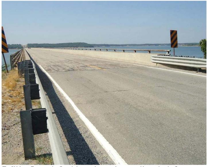
The Oklahoma Transportation Commission recently approved a contract with an engineering firm to prepare construction plans for replacement of the SH-99/US-377 bridge near Willis, just south of Madill in Marshall County. The bridge spans Lake Texoma and is the largest structurally deficient bridge in the state.
