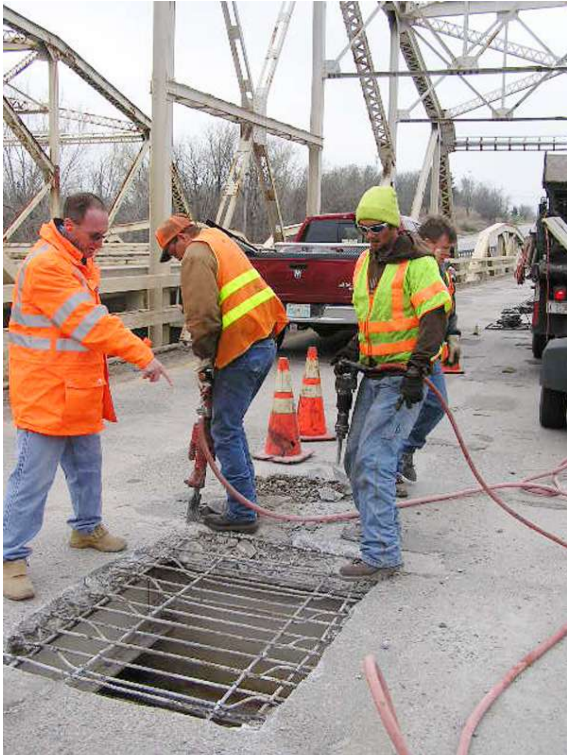
One of 40: ODOT crews make an emergency repair to the SH-66 bridge over Bird Creek in Rogers County. The repair was one of more than 40 emergency repairs made in the last three years. On Monday, Dec. 6, members of the Oklahoma Transportation Commission approved a contract to build detours around the bridge until it can be replaced next fall.
