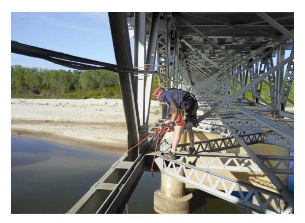
An ODOT engineer inspects a series of gusset plates, or connectors, on the US-77 bridge between Lexington and Purcell. Although truss bridges in Oklahoma have been inspected three times since the Minnesota bridge collapse, ODOT officials ordered a review of gusset plate design after a federal study indicated the connectors played a role in the tragedy. Gusset plates were used in construction of truss bridges, which were built on state highways until the mid-1960s. About 95 such bridges remain.
