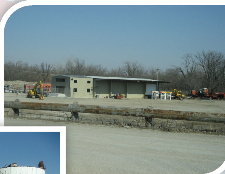
Concrete Recycling Center:
