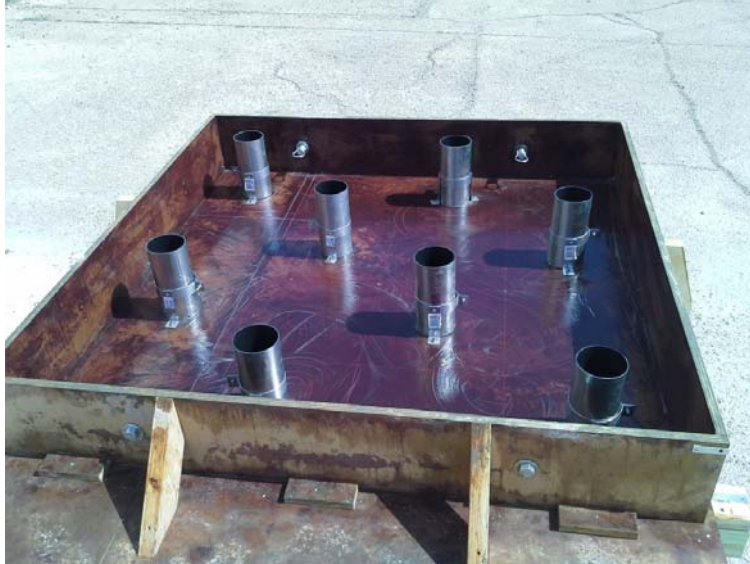
Figure 3: Formwork with cast-in-place cylinder holders fixed.
