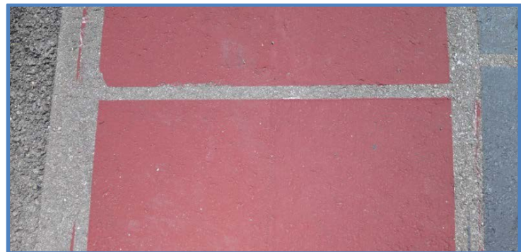
Figure 7. ULTRASEAL® containing red pigment applied to existing asphalt surface
