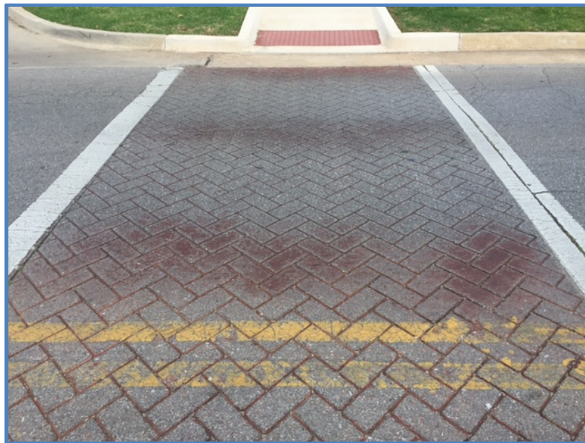
Figure 12. Asphalt containing red pigment used to delineate pedestrian crosswalk
