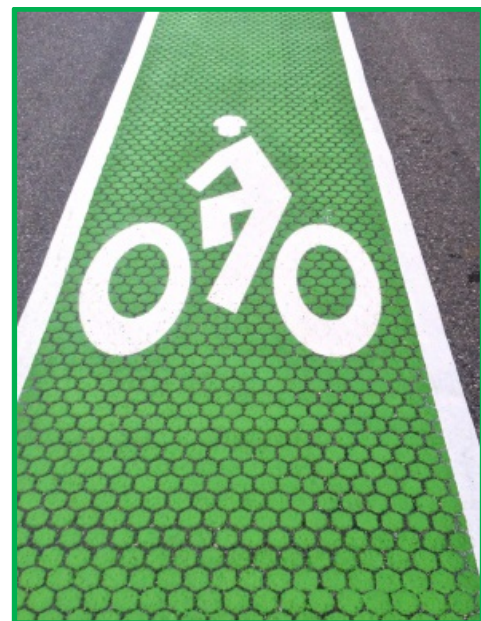
Figure 5. Portland Cement Slurry Surfacing used in New Jersey
