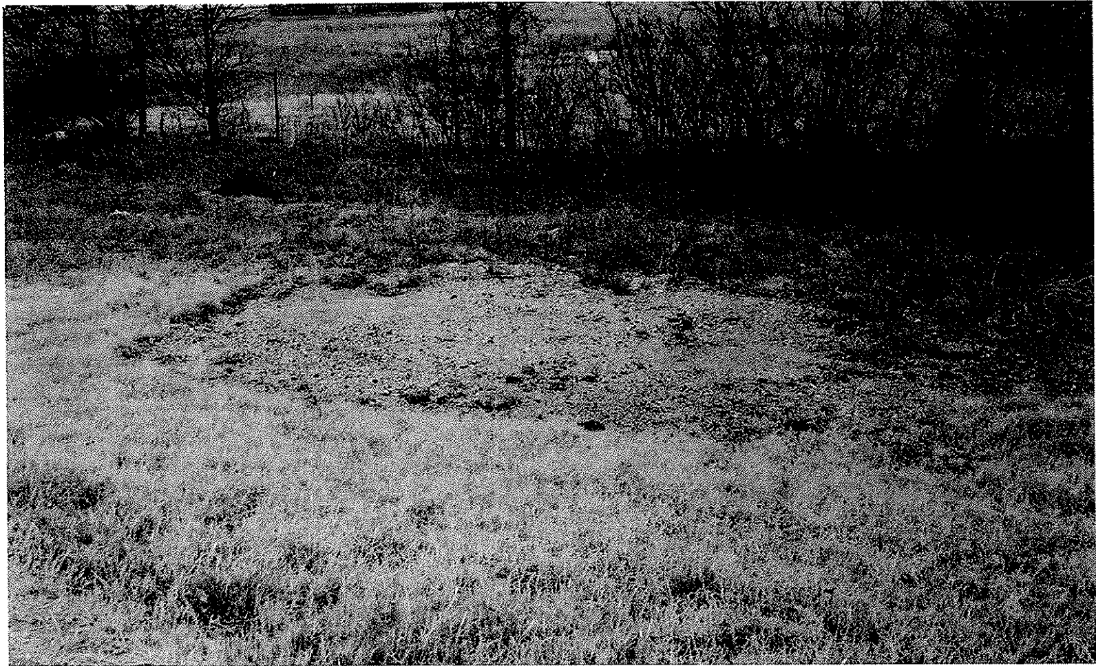
Figure 7. Looking North Across New Sinkhole July 2003.
