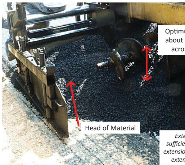
Optimum amount of mix should cover about 75% of the height of the augers across the full width of the screed
