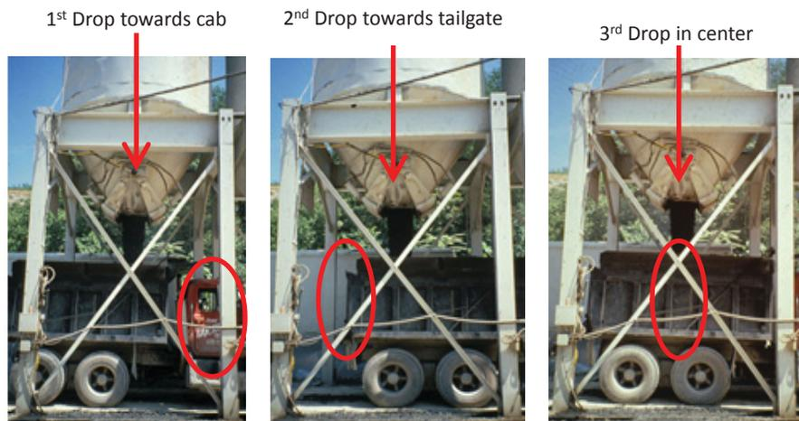
FIGURE 45 Loading with multiple drops [Source: Scherocman (2011)].
