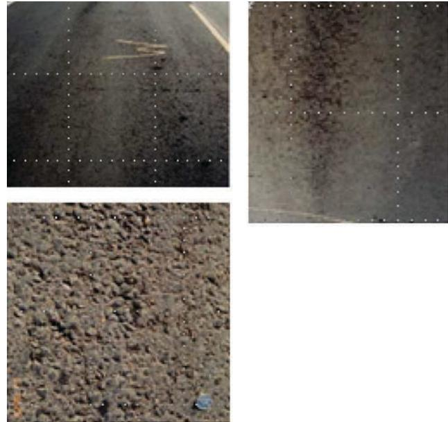
FIGURE 10 Example of moderate level of segregation [Source: Gavin and Heath (2002)].
