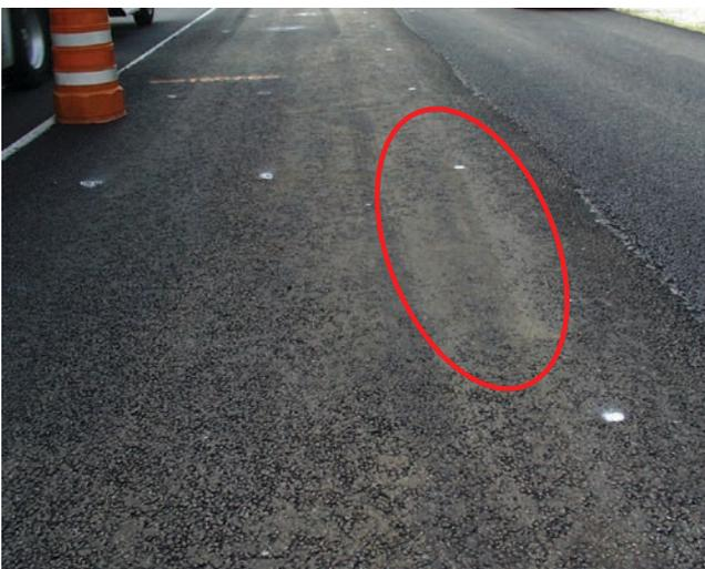
FIGURE 5 Example of random segregation (separation of binder and stone) in SMA [Source: Stroup-Gardiner (2014)].
