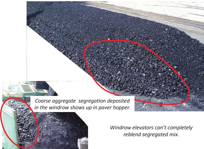
*Coarse aggregate segregation deposited in the windrow shows up in paver hopper.*
