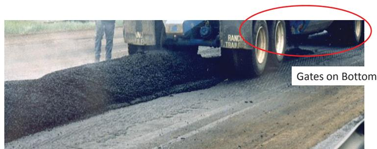
Belly dumps drop mix when the gates at the bottom of the truck bed deposit mix into a windrow on the exiting surface
