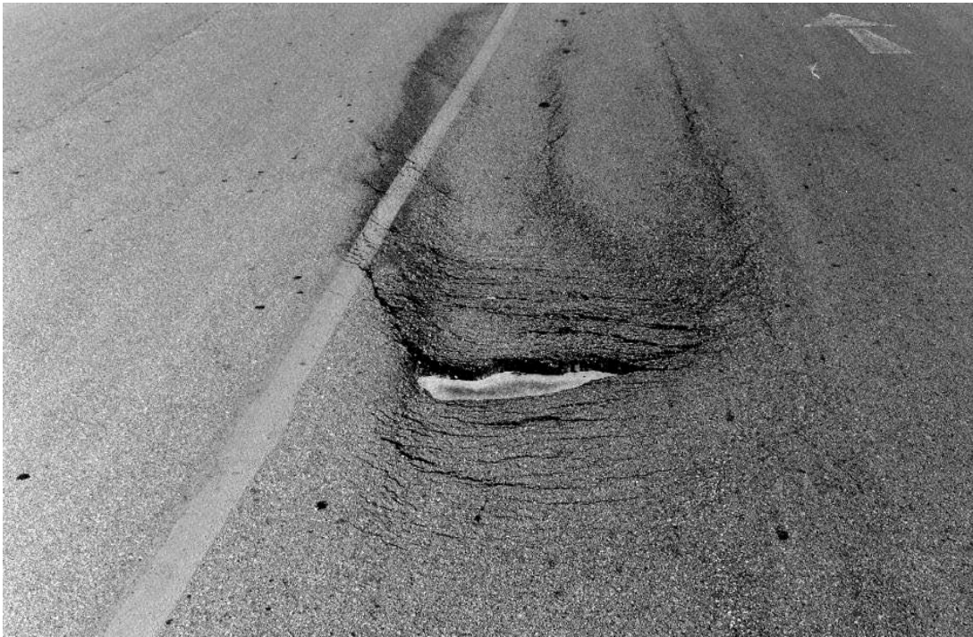
Figure 1. Slippage failure due to poor bonding of pavement layers.
