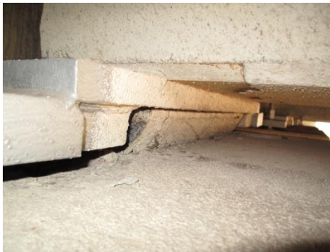
Figure 1. 19th Street Bridge (I-35 under) in Moore, OK. (a) Distresses on bridge abutment (b) Shearing of elastomeric bearings
