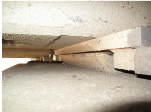
Figure 1. 19th Street Bridge (I-35 under) in Moore, OK. (a) Distresses on bridge abutment (b) Shearing of elastomeric bearings
