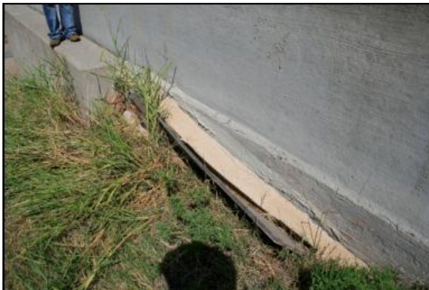
Figure 12 Maintenance Under Approach Slab
