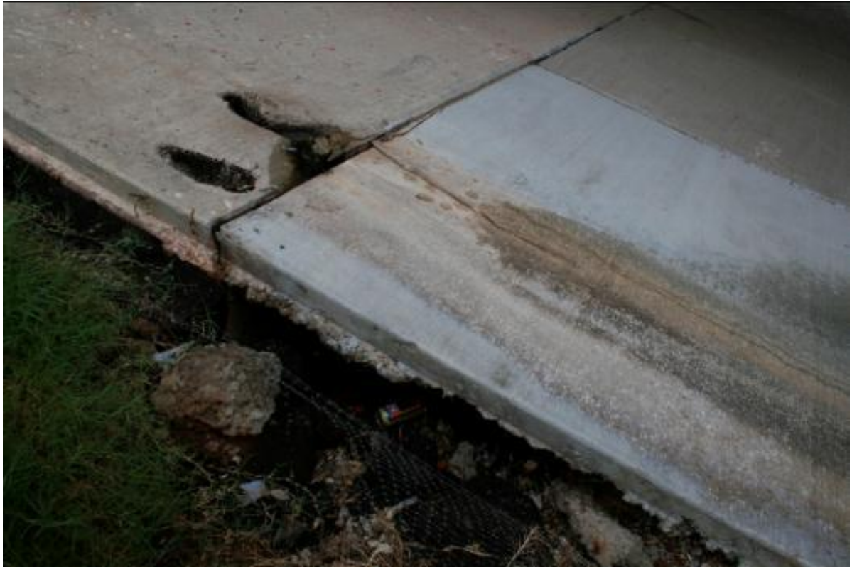
Figure 10 Drains and Voids At Slope Wall
