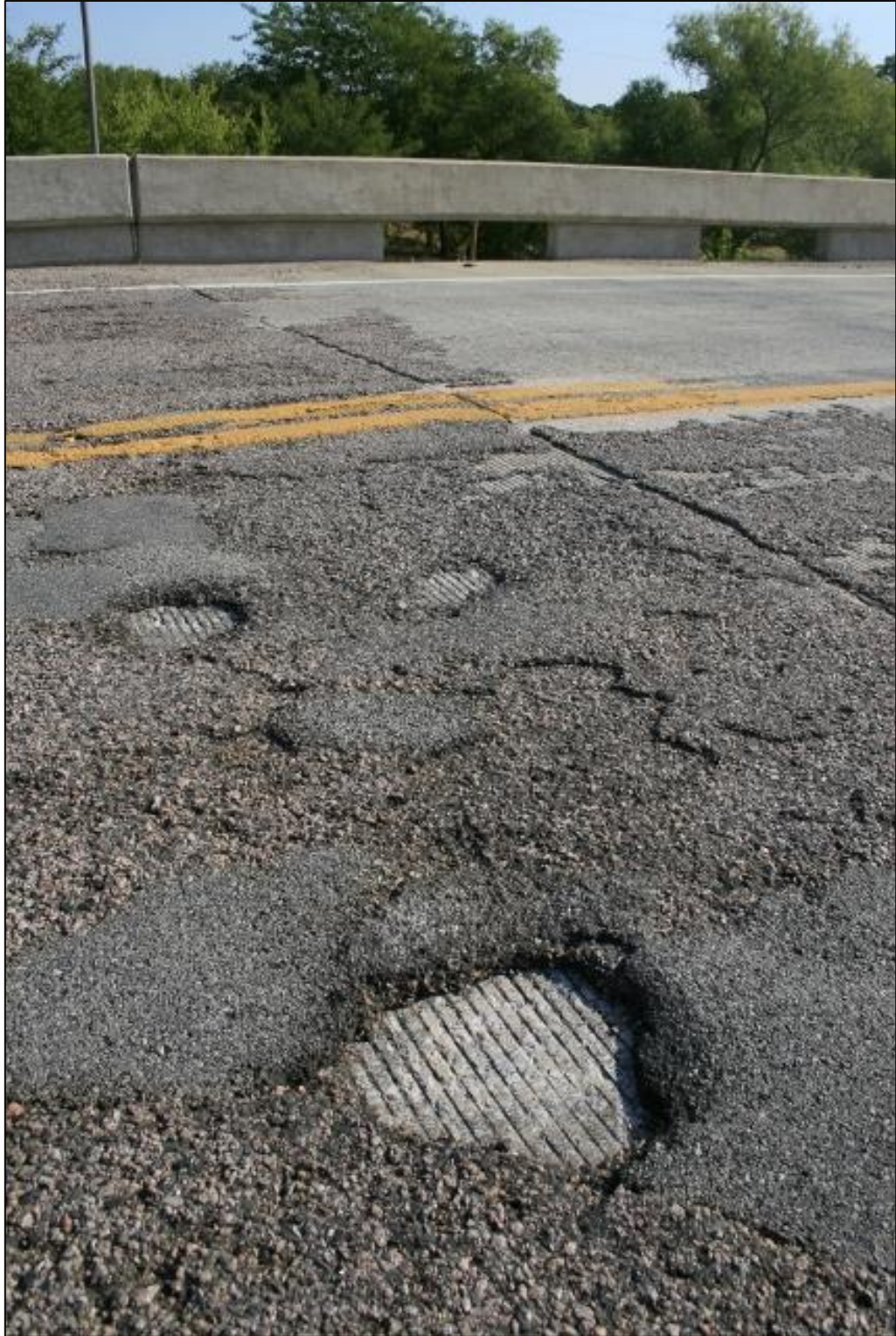
Figure 16 Asphalt Over Concrete, Approximately 2" Thick
