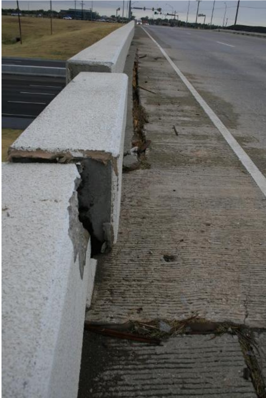
Figure 7 Horizontal Displacement; Looking West Across Tecumseh Road Bridge
