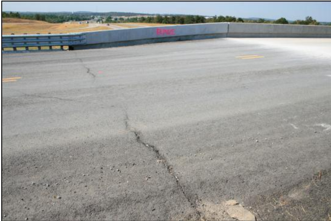
Figure 17 Hereford Lane East Approach: Pre-Demolition
