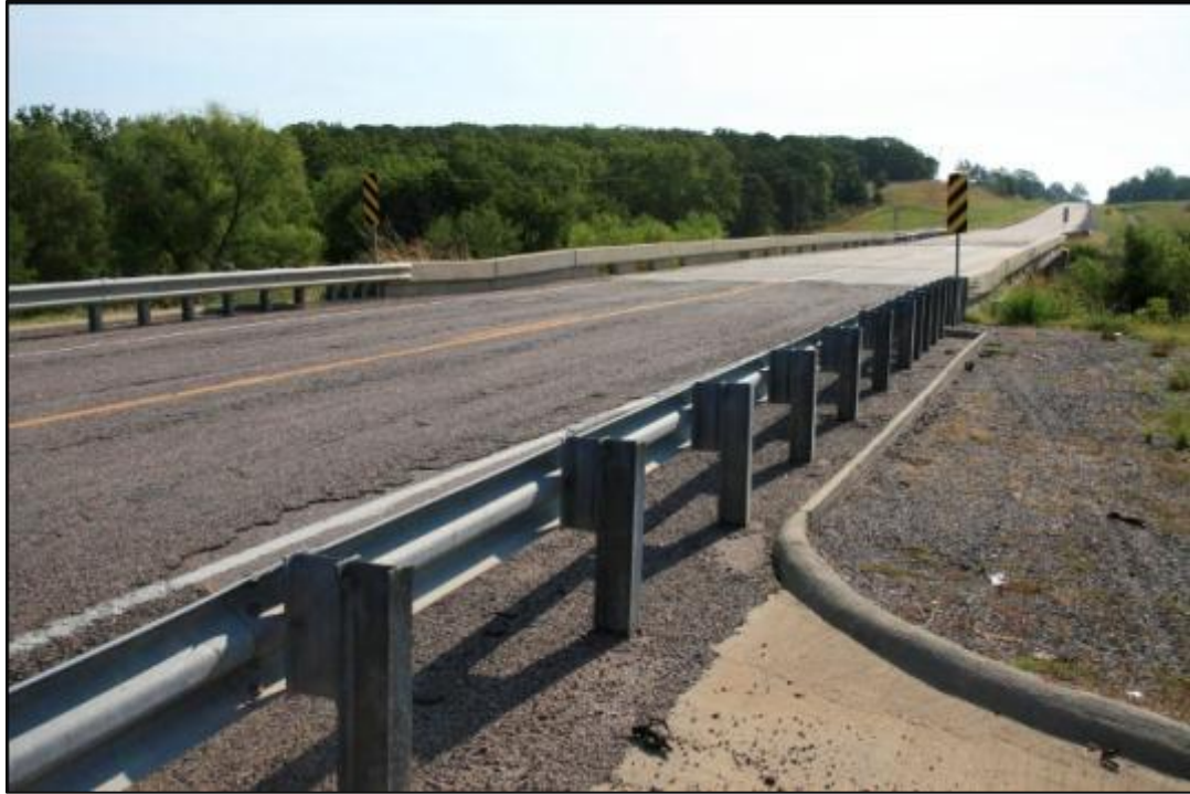
Figure 13 Overview of Site
