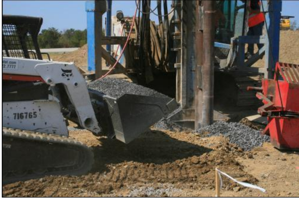
Figure 21 Placing and Vibrating Aggregate
