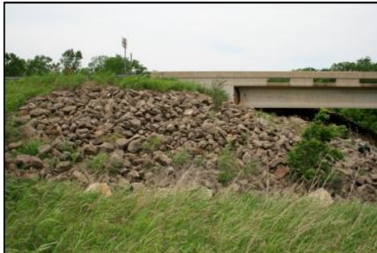
Figure 3 US 177 Embankment A-1
