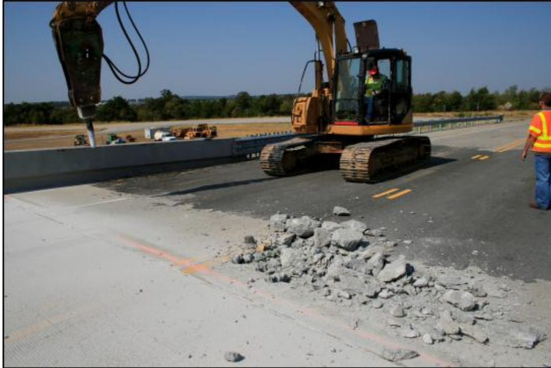
Figure 18 Hereford Lane West Approach: Demolition
