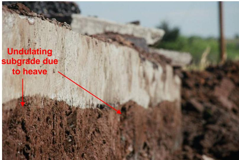
**Figure 2-5: Cross-section of Highway 412 in Woodward, OK from Dr. Jim Nevels**
