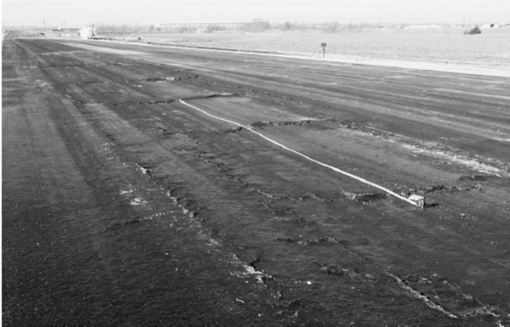
**Figure 2-4.** Sulfate Heave on U.S. 67 in Waxahachie, TX from Harris et al. 2003
