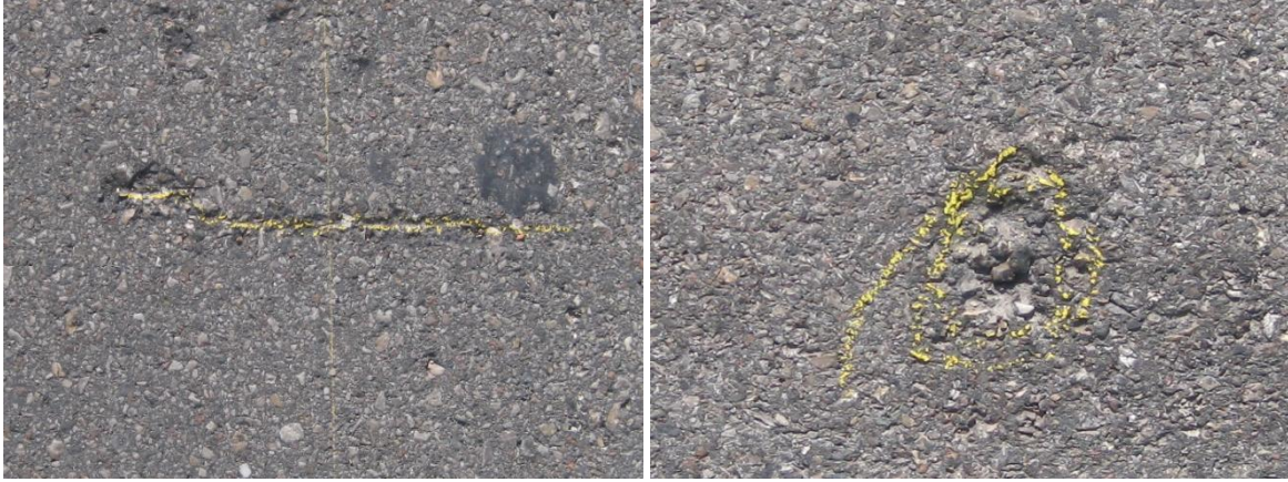
Figure 3: Photographic View of Loss of Aggregates from Pavement at a Distance of (a) 318 ft and (b) 741 ft from North End of the Test Section
