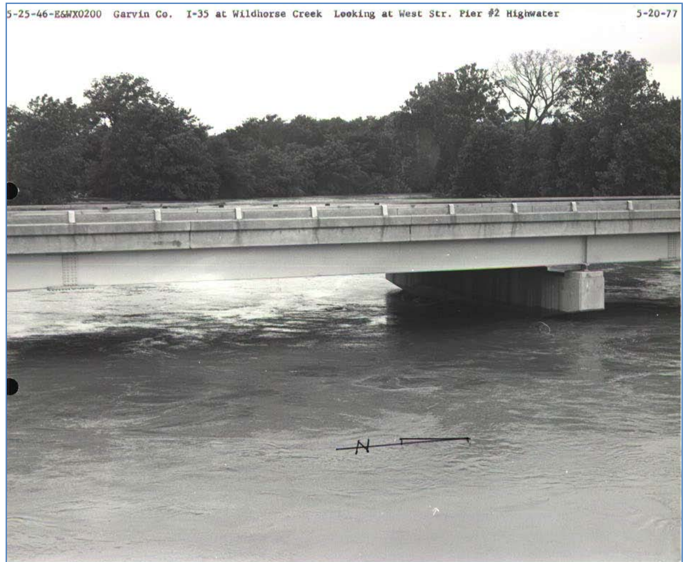
Figure 24. Picture demonstrating flood water level at pier at bridge 17590 on I-35 NB over Wildhorse Creek.
