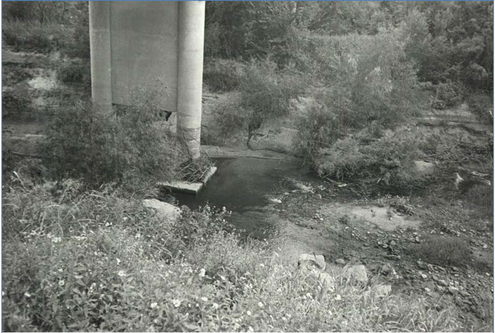
Figure 22. Picture demonstrating extent of damage to pier ar bridge 12643 on SH 76 over Rush Creek.
