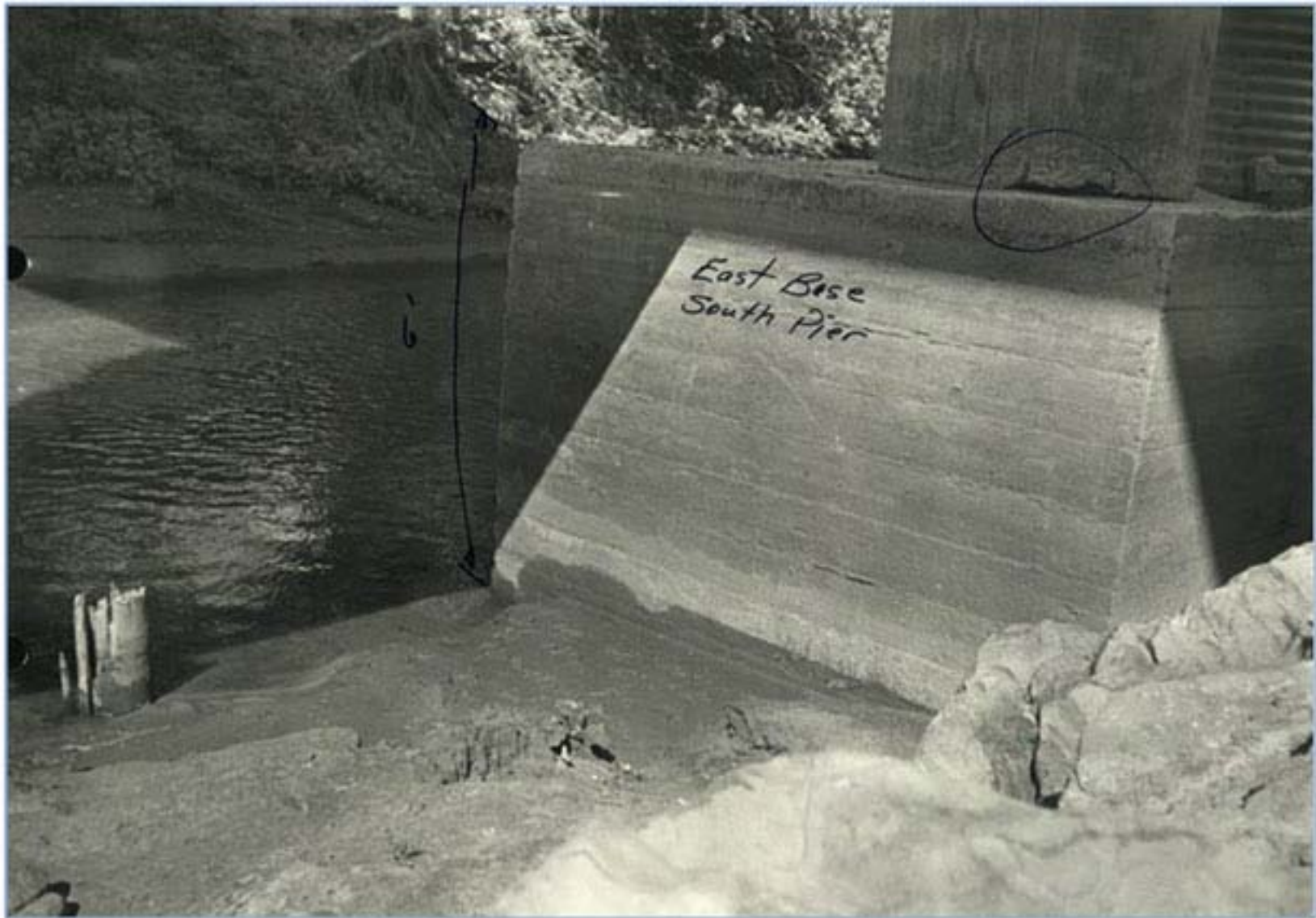
Figure 20. Picture demonstrating extent of damage to south pier at bridge 10738 on SH 74 over Rush Creek.
