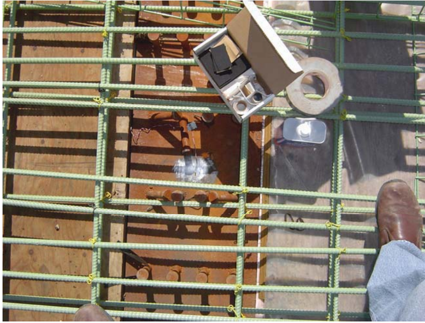
Strain Gauge mounted and ready for protective coatings
