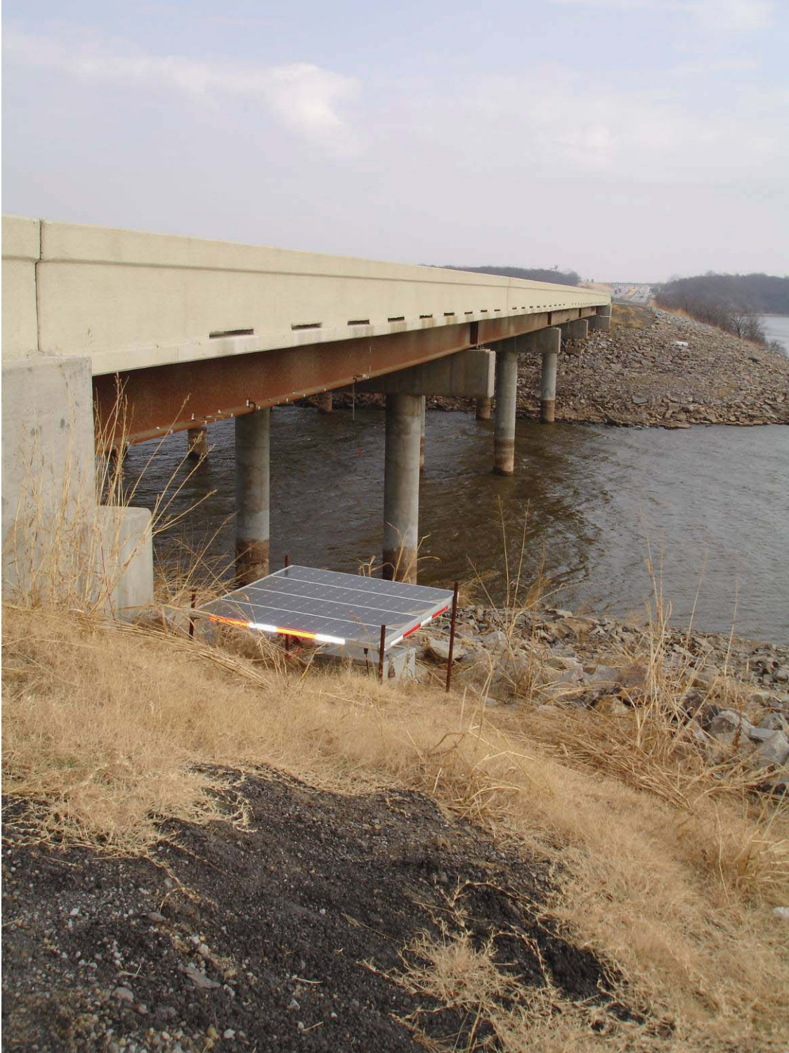
Solar collector powering data collection system – Jan. 2006
