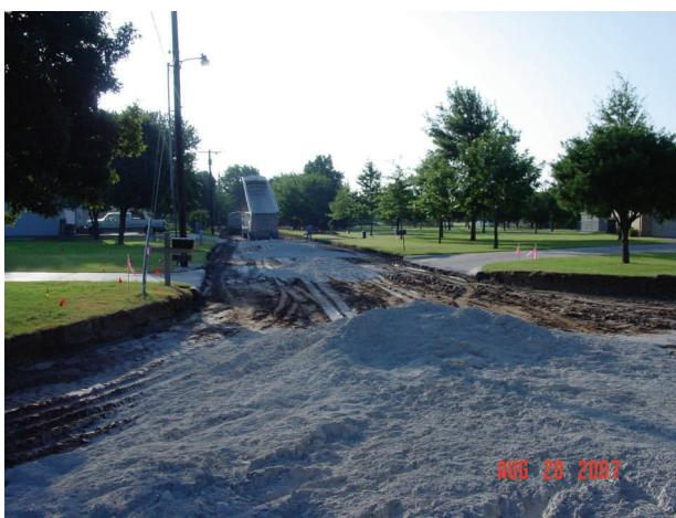
Questions arise with regard to chemically treated subgrade soils about the rate of development and ultimate magnitude of improvement (strength increase or volume change stability) on construction projects. In other words, is the improvement response of field constructed soil layers the same as the laboratory mix design response? Potential
