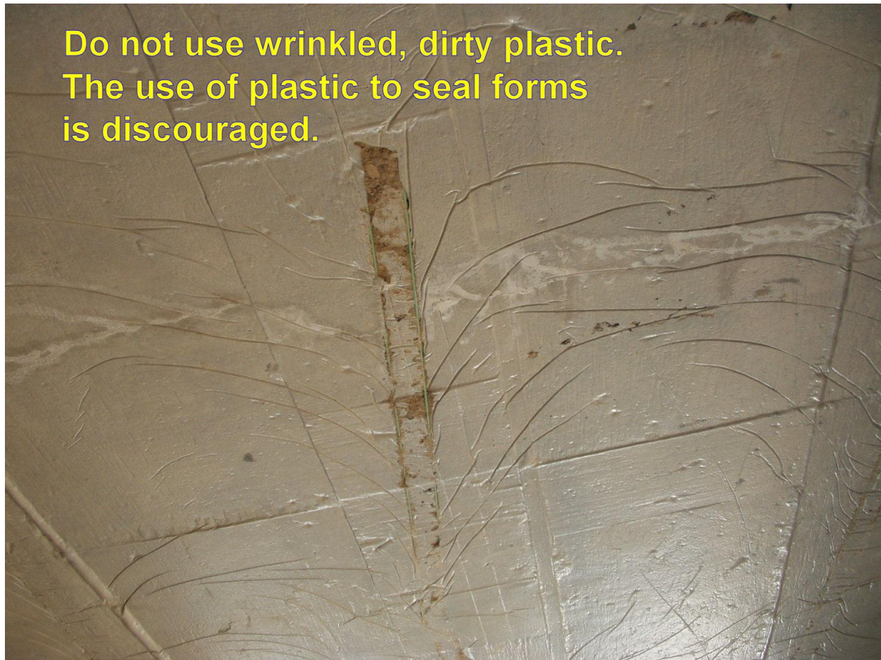
Figure 504:1. Photo. Sealing Forms with Plastic
