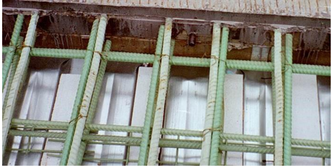
Figure 511:1. Photo. Unacceptable Exposure of Epoxy Coated Steel
