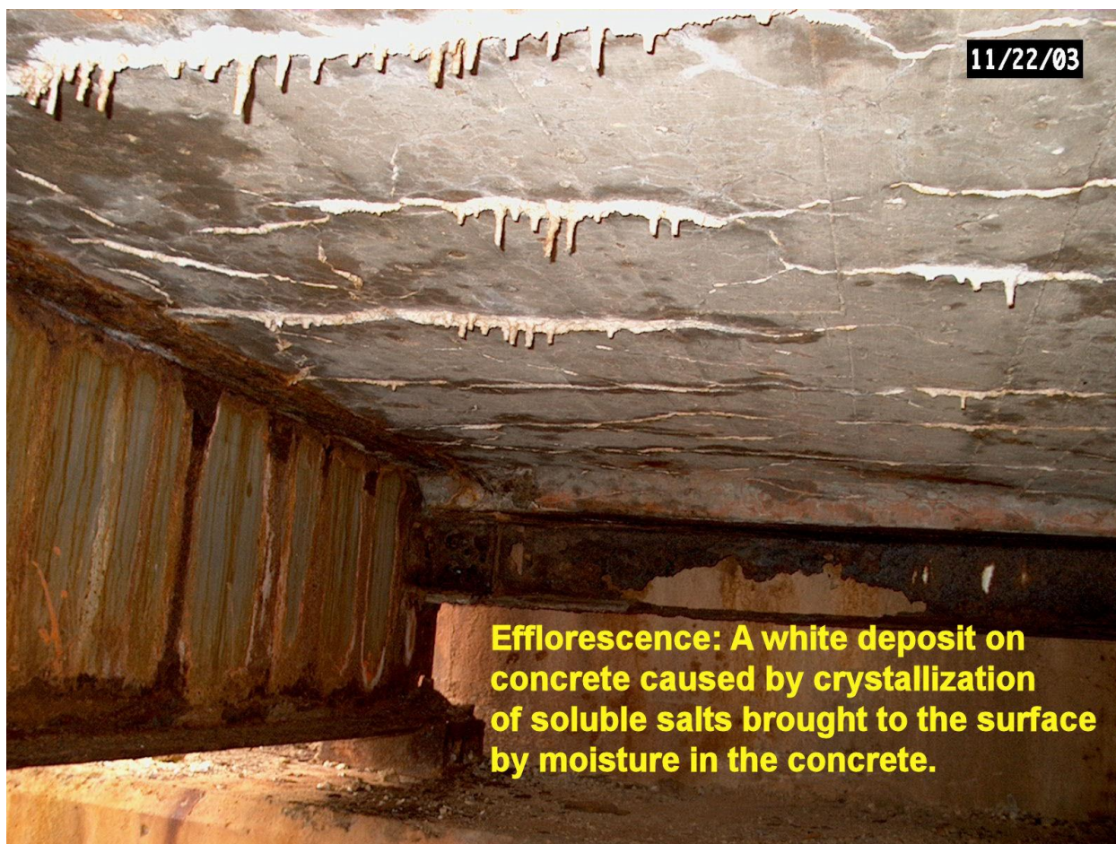
Figure 520:1. Photo. Efflorescence
