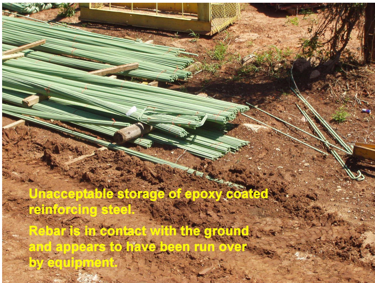
Figure 511:2. Photo. Unacceptable Storage of Epoxy Coated Steel
