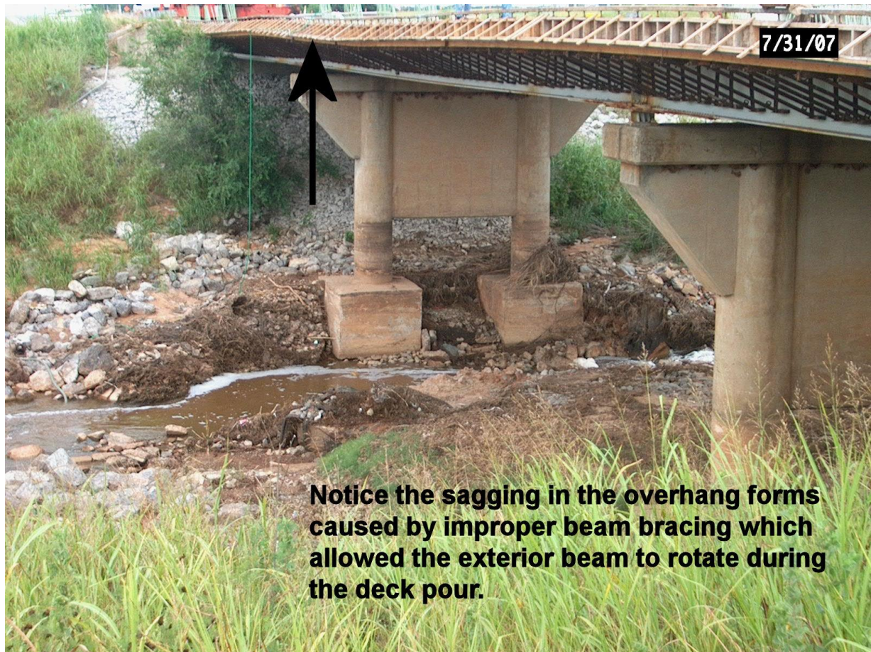
Figure 506:8. Photo. Sagging due to Inadequate Beam Bracing
