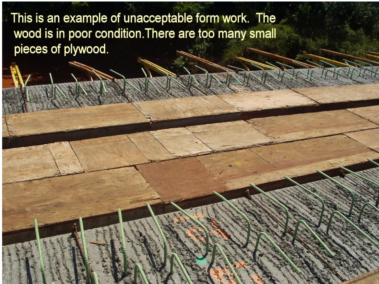
Figure 502:2. Photo. Unacceptable Form Work
