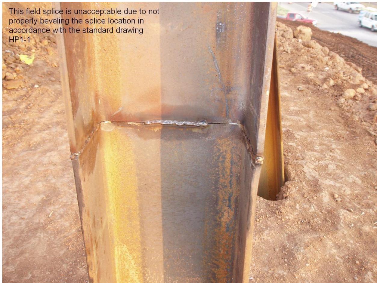
Figure 514:3. Photo. Unacceptable Field Splice
