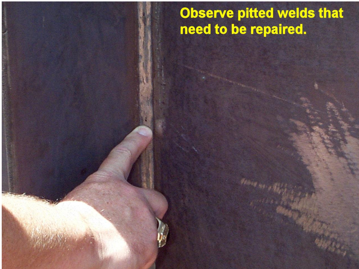
Figure 506:3. Photo. Pitted Welds in need of Repair
