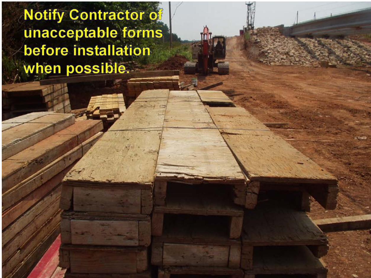
Figure 502:3. Photo. Unacceptable Forms
