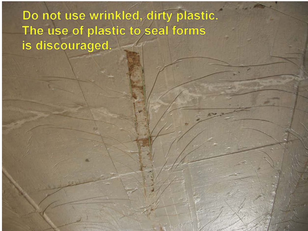
Figure 504:1. Photo. Sealing Forms with Plastic
