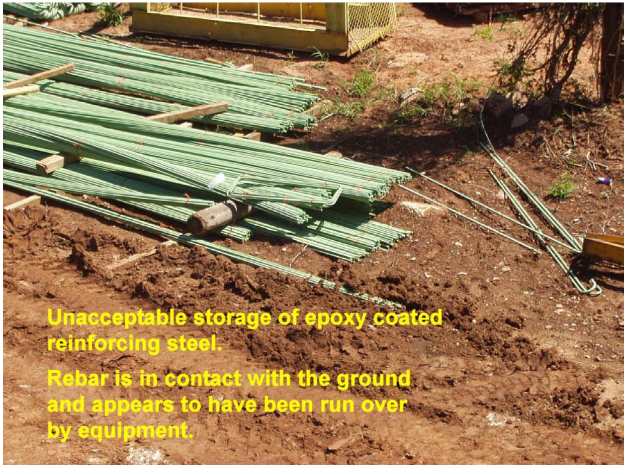
Figure 511:1. Photo. Unacceptable Storage of Epoxy Coated Steel
