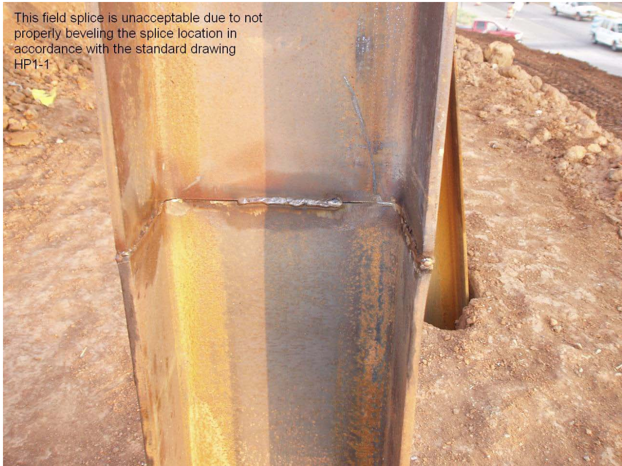
Figure 514:3. Photo. Unacceptable Field Splice
