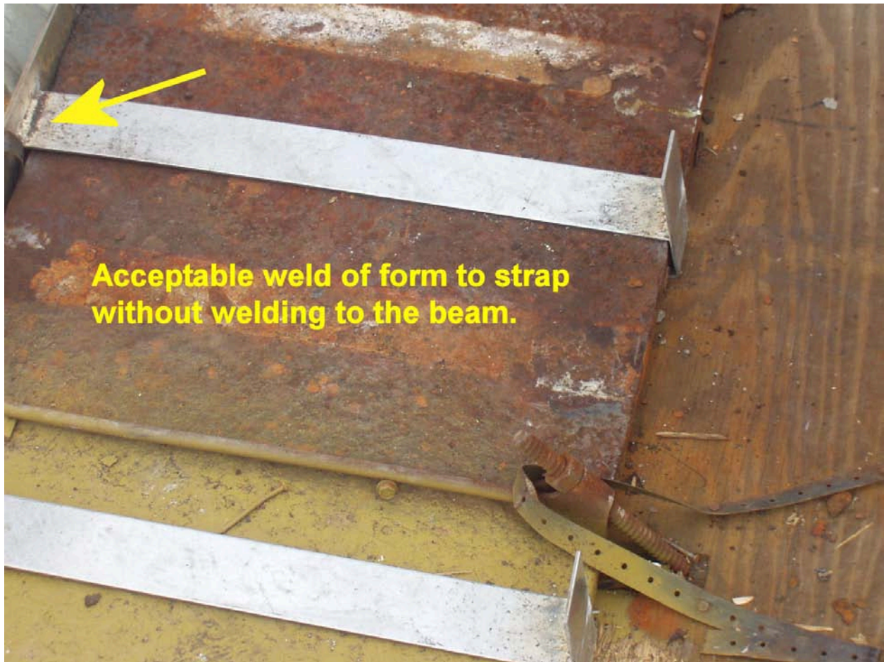
Figure 502:6. Photo. Acceptable Weld of Stay-in-Place Forms
