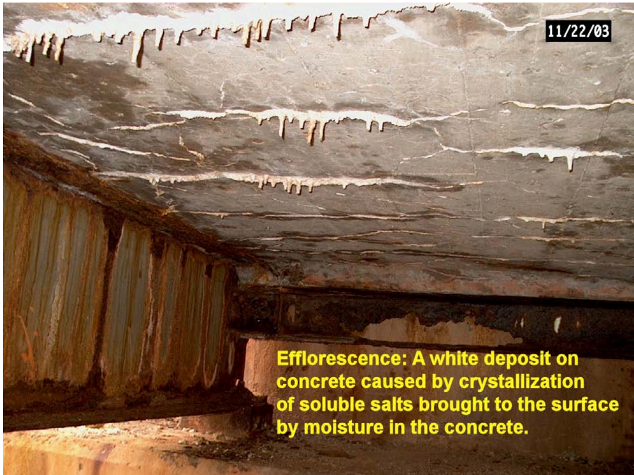
Figure 520:1. Photo. Efflorescence
