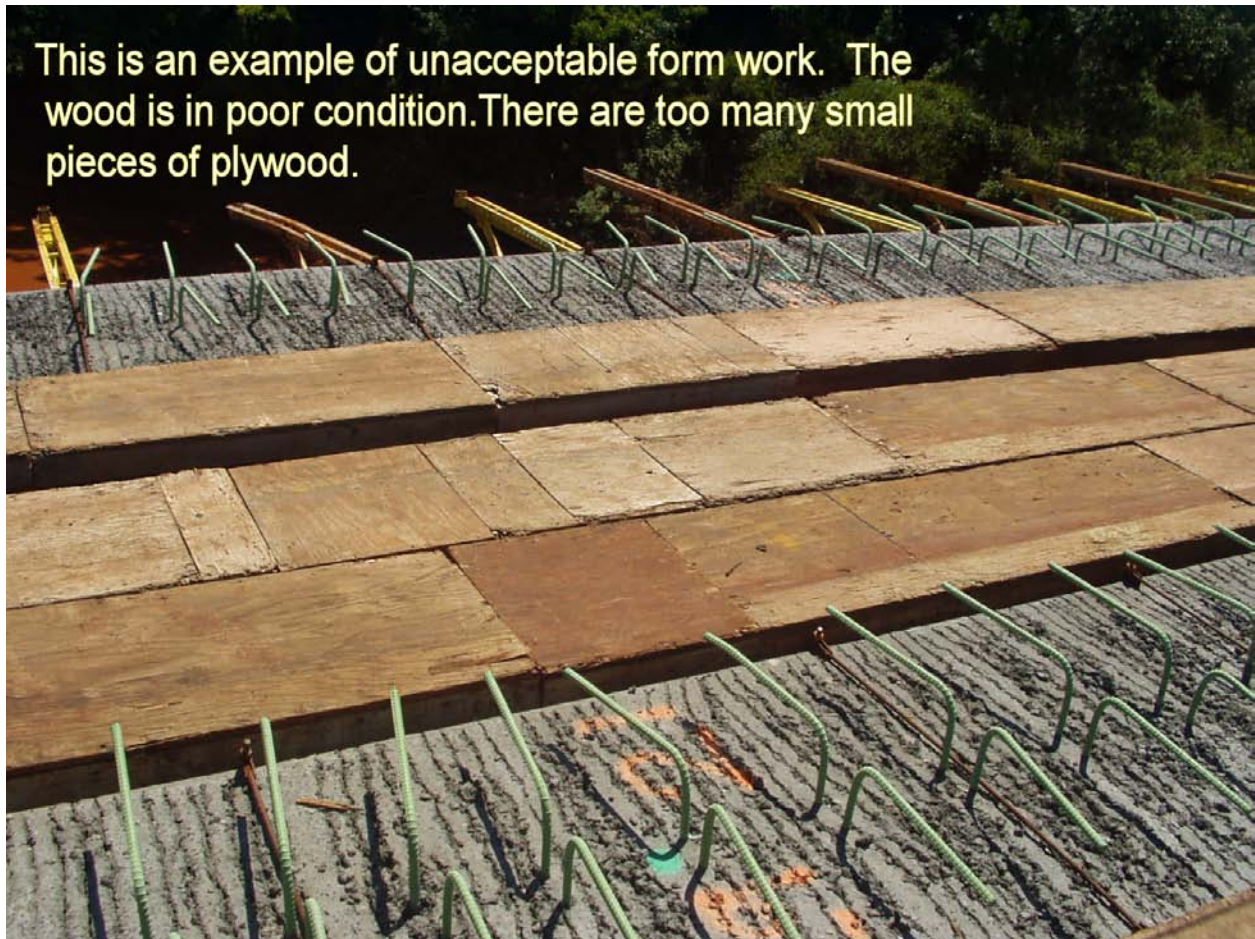
Figure 502:2. Photo. Unacceptable Form Work
