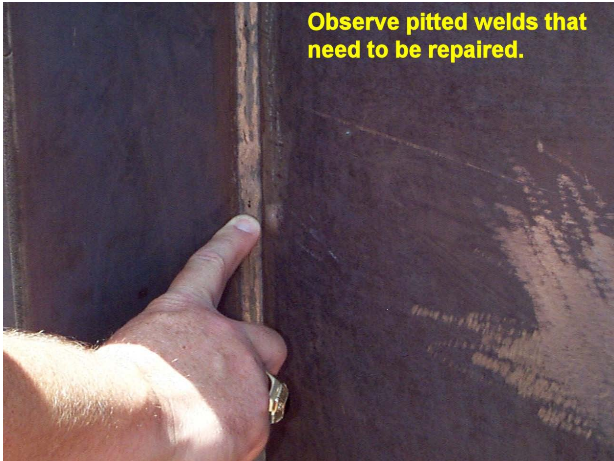
Figure 506:3. Photo. Pitted Welds in need of Repair
