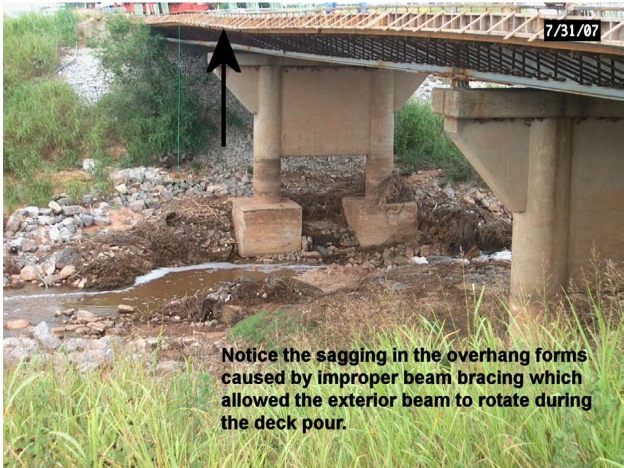
Figure 506:8. Photo. Sagging due to Inadequate Beam Bracing
