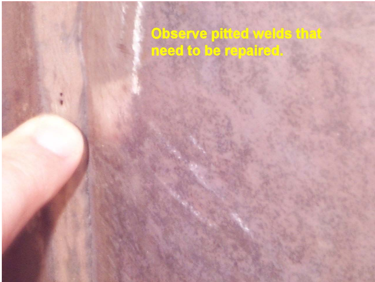
Figure 506:4. Photo. Pitted Welds in need of Repair
