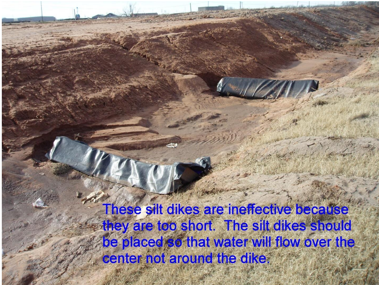
Figure 221:4. Photo. Ineffective Silt Dikes
