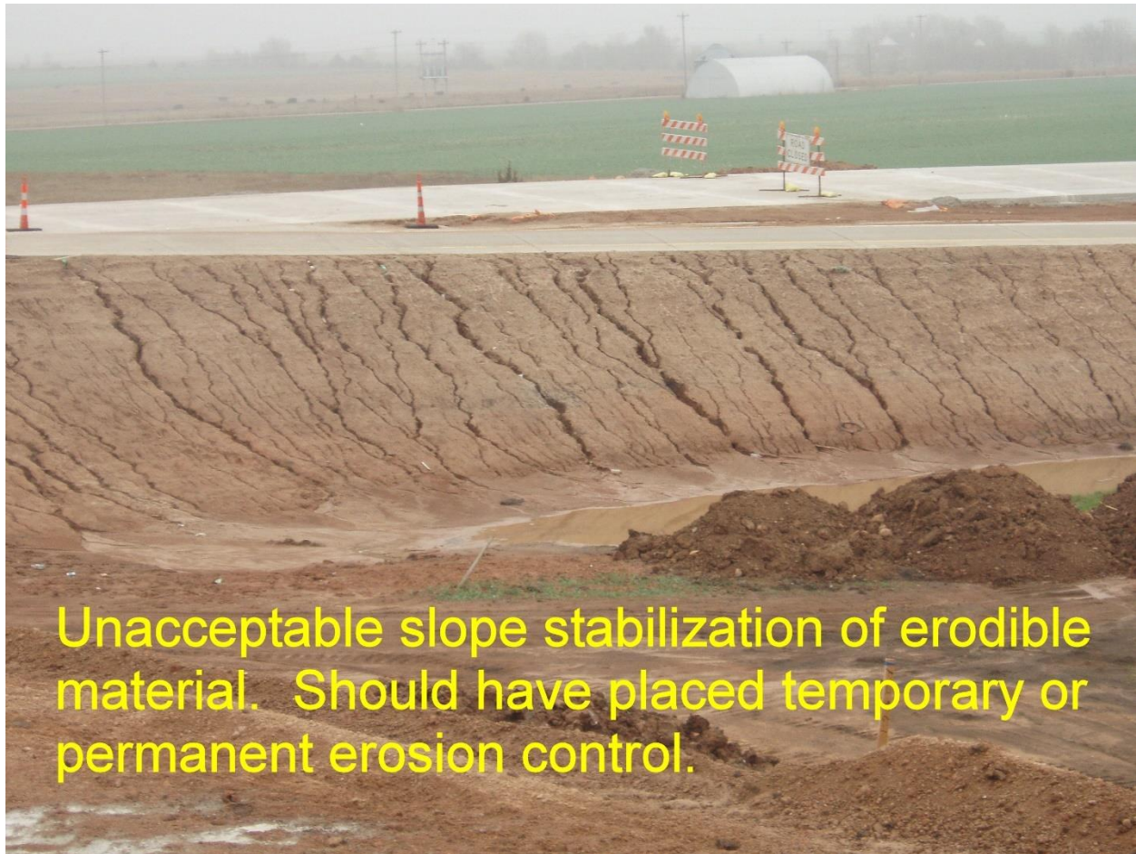
Figure 220:4. Photo. Unacceptable Slope Stabilization
