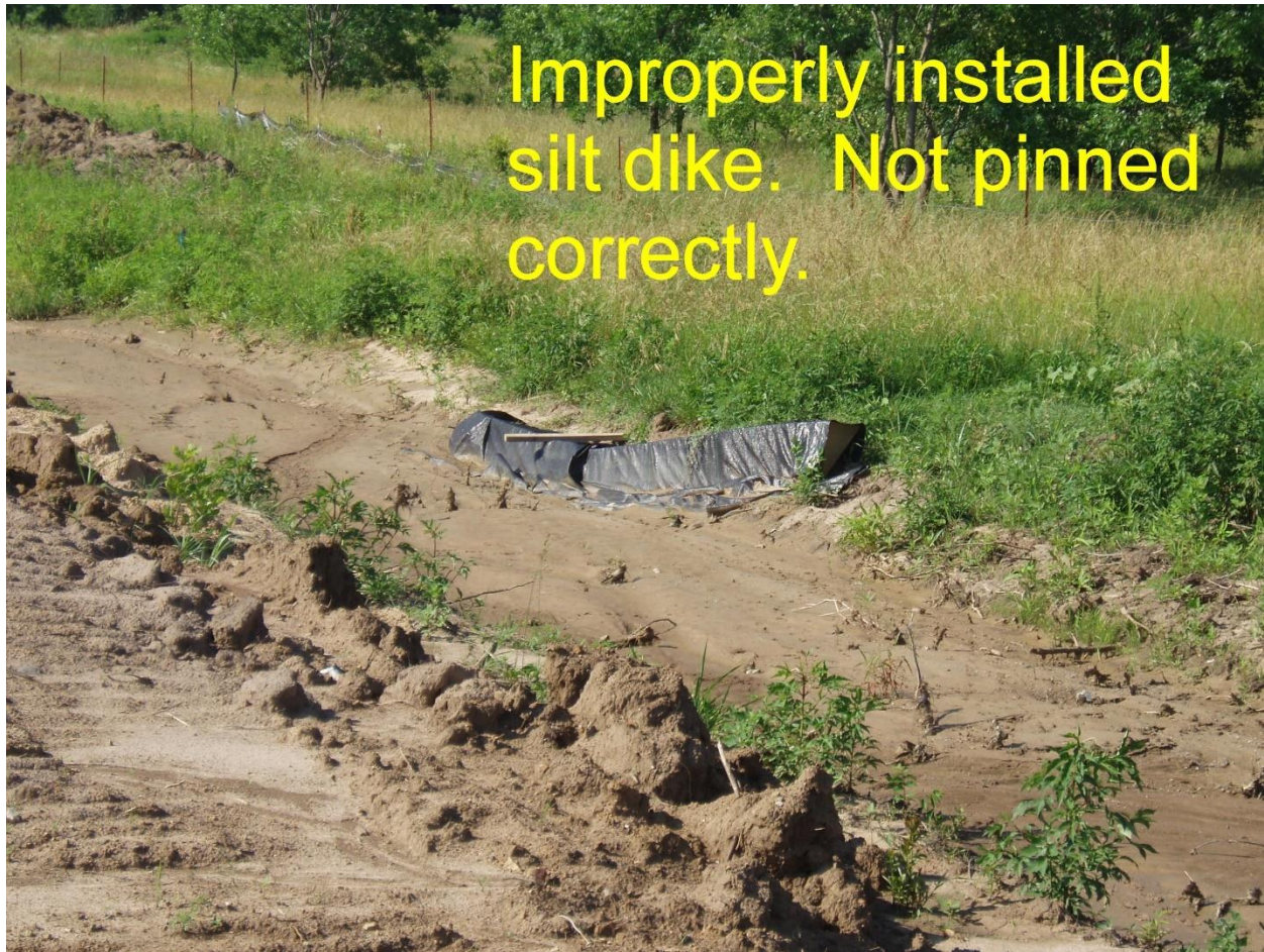
Figure 221:3. Photo. Improperly Installed Silt Dike
