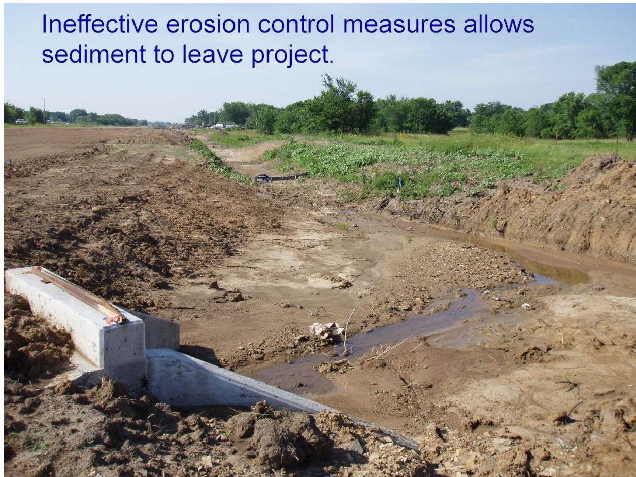
Figure 220:1. Photo. Ineffective Erosion Control Measures
