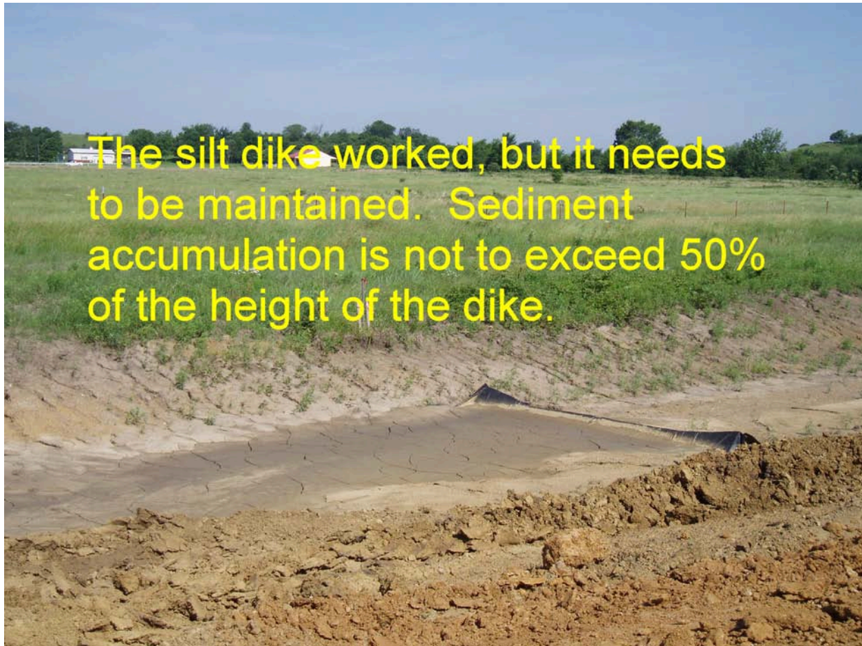
Figure 221:5. Photo. Inadequate Maintenance of Silt Dike
