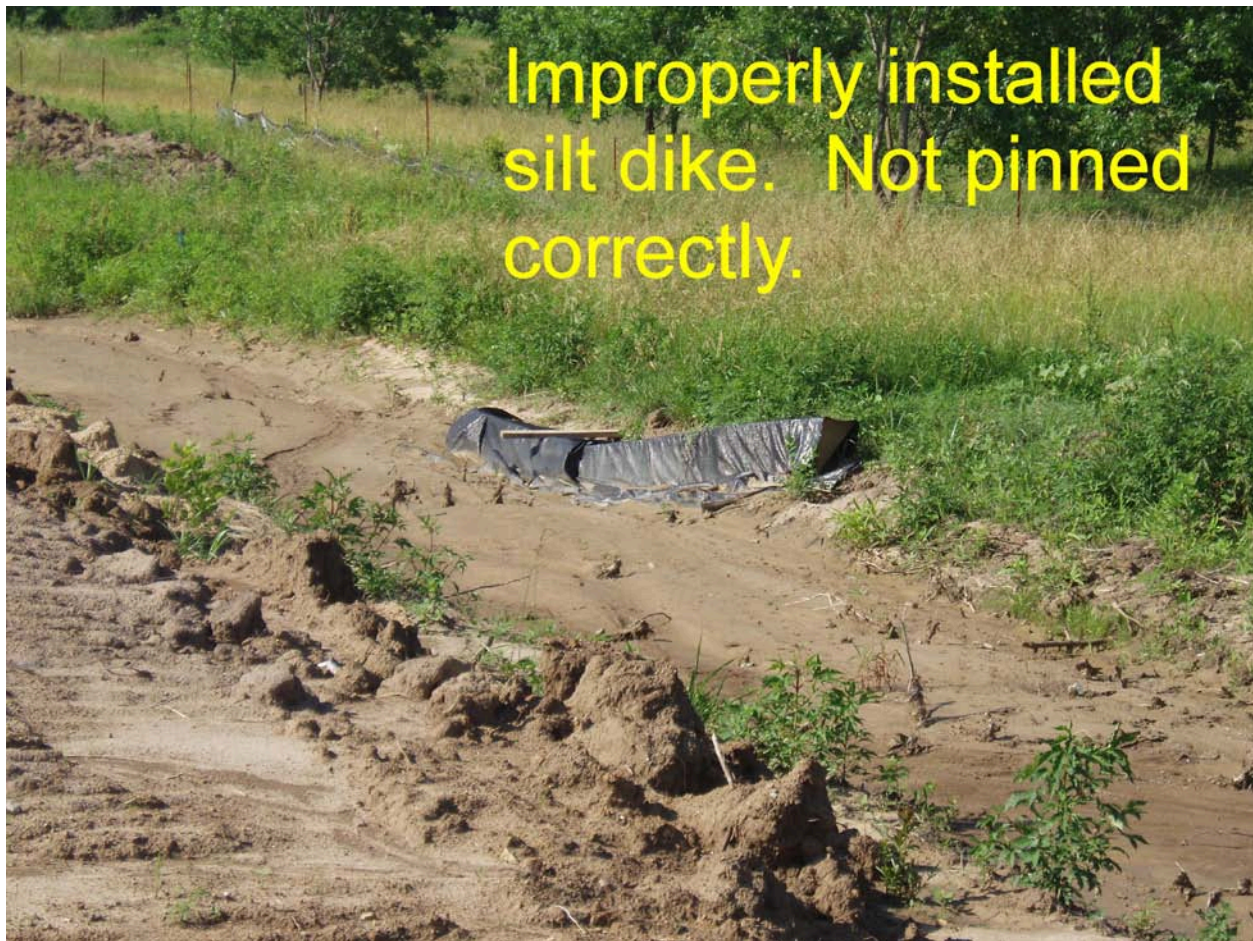
Figure 221:3. Photo. Improperly Installed Silt Dike
