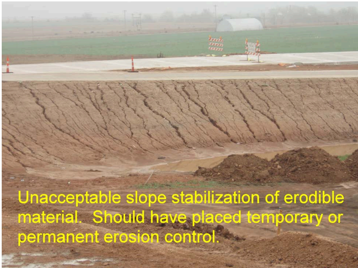
Figure 220:4. Photo. Unacceptable Slope Stabilization
