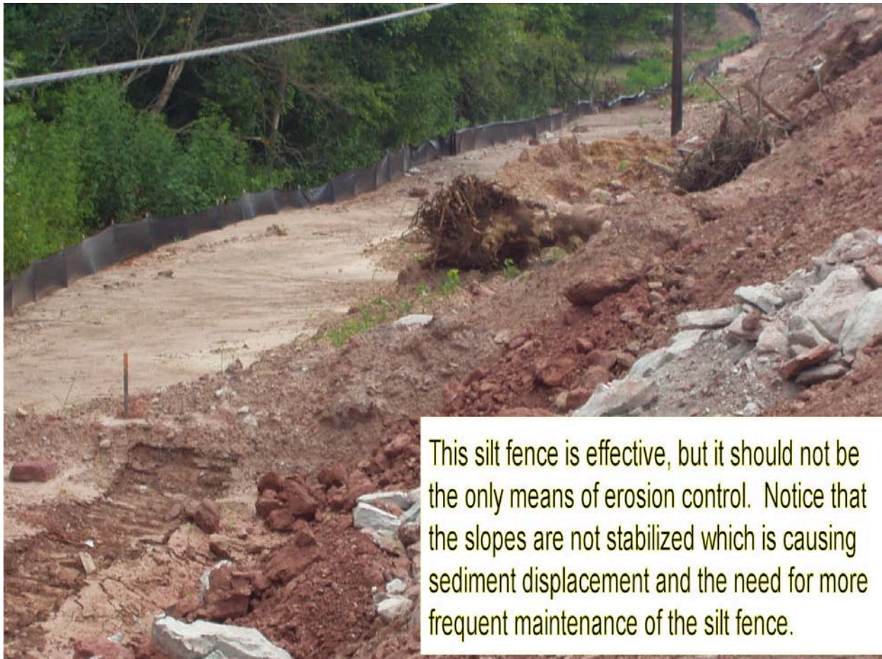
Figure 221:1. Photo. Silt Fence
