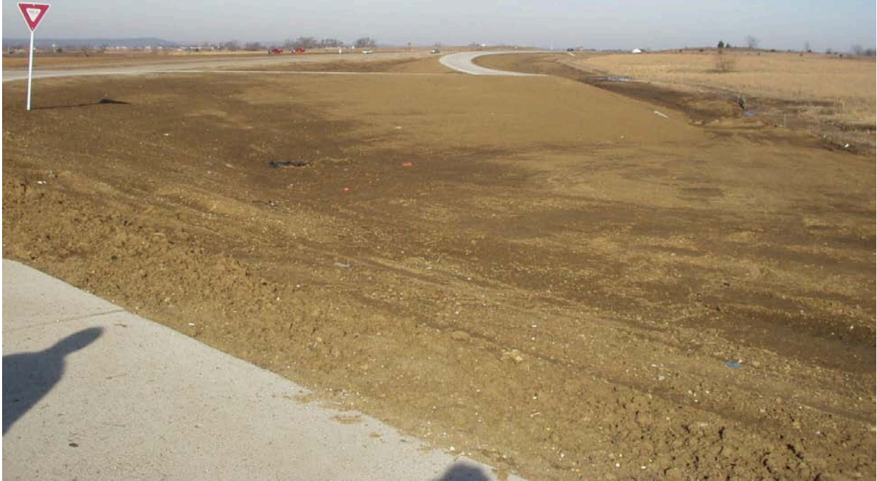
Figure 220:2. Photo. Completed Slope Prior to Stabilization
