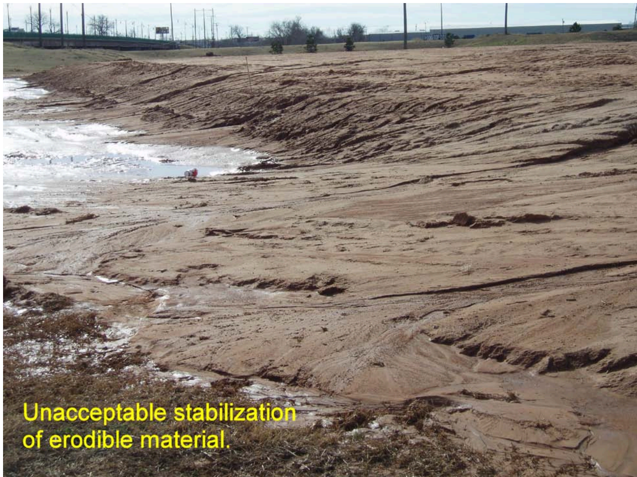
Figure 220:5. Photo. Unacceptable Stabilization of Erodible Material
