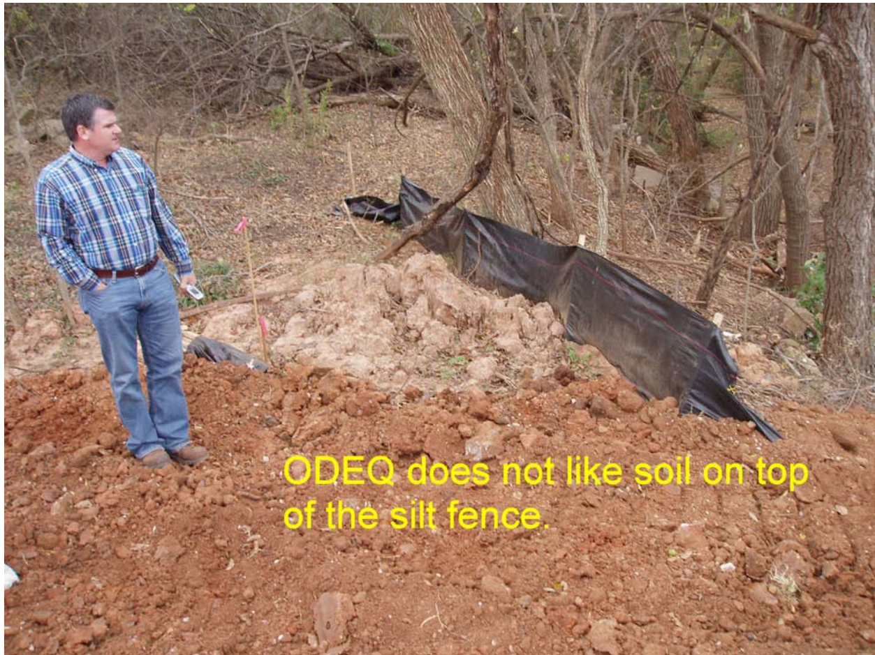
Figure 221:2. Photo. Inadequate Maintenance of Silt Fence
