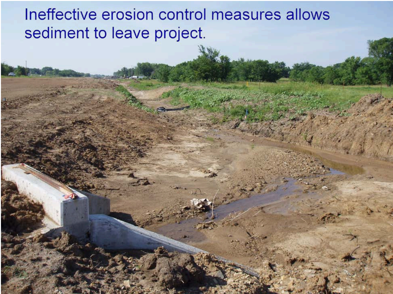
Figure 220:1. Photo. Ineffective Erosion Control Measures
