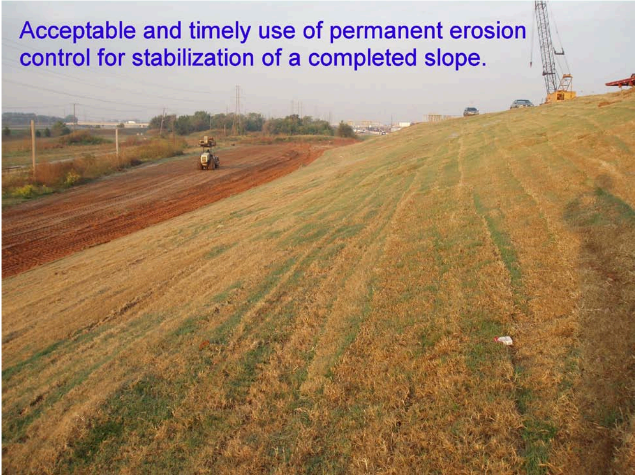
Figure 220:3. Photo. Proper Stabilization of a Completed Slope
