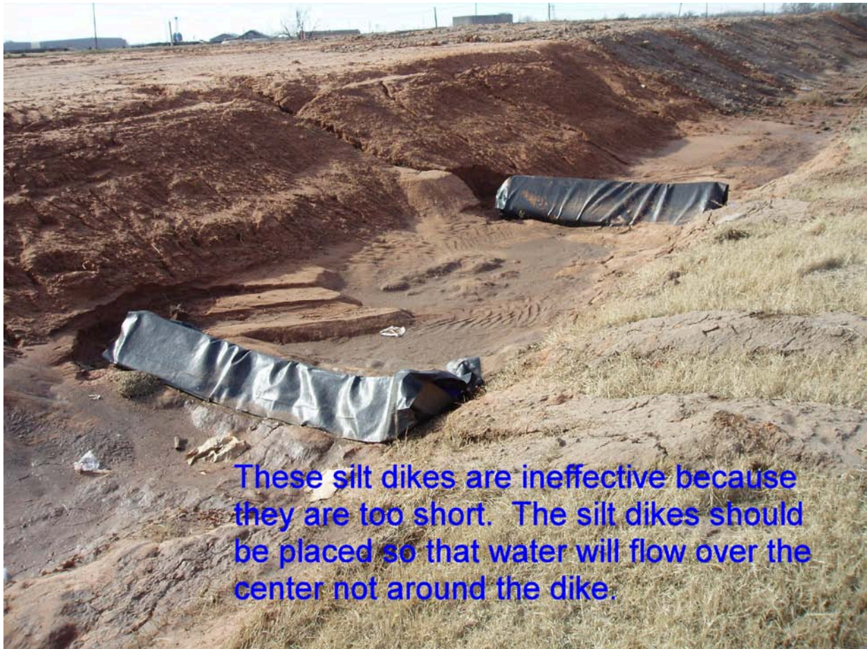
Figure 221:4. Photo. Ineffective Silt Dikes
