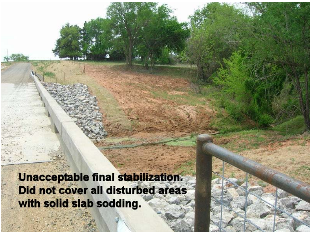
Figure 220:6. Photo. Unacceptable Final Stabilization
