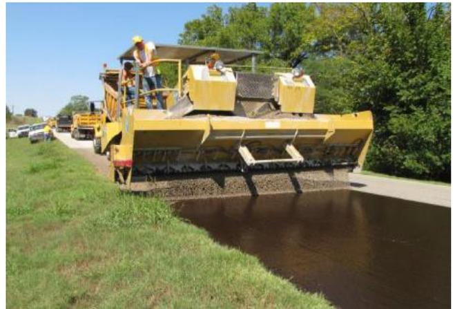
**Figure 1 Chip Seal Installation on SH39**
