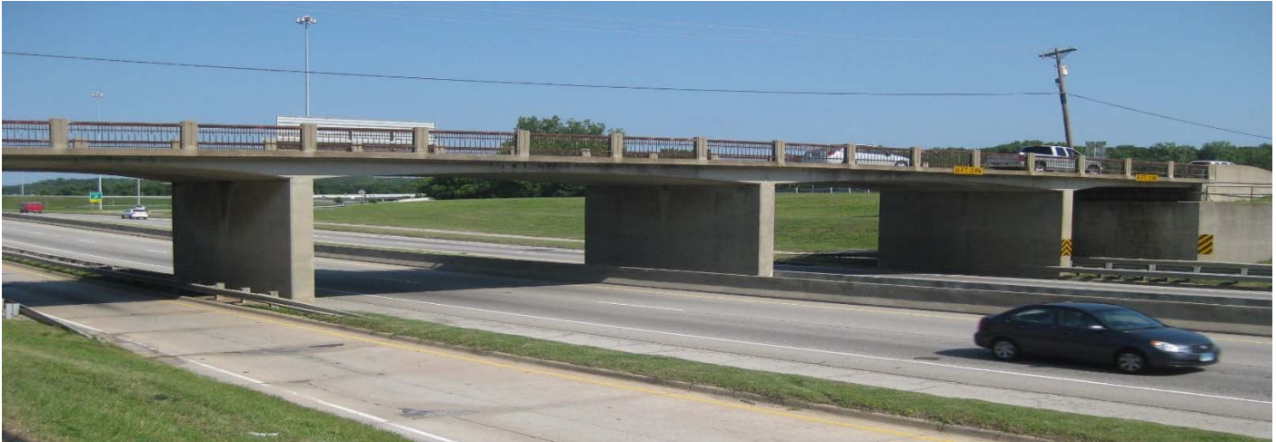
FIGURE 2. Bridge on Union Avenue over I-44 from 1952 - Functionally Obsolete
