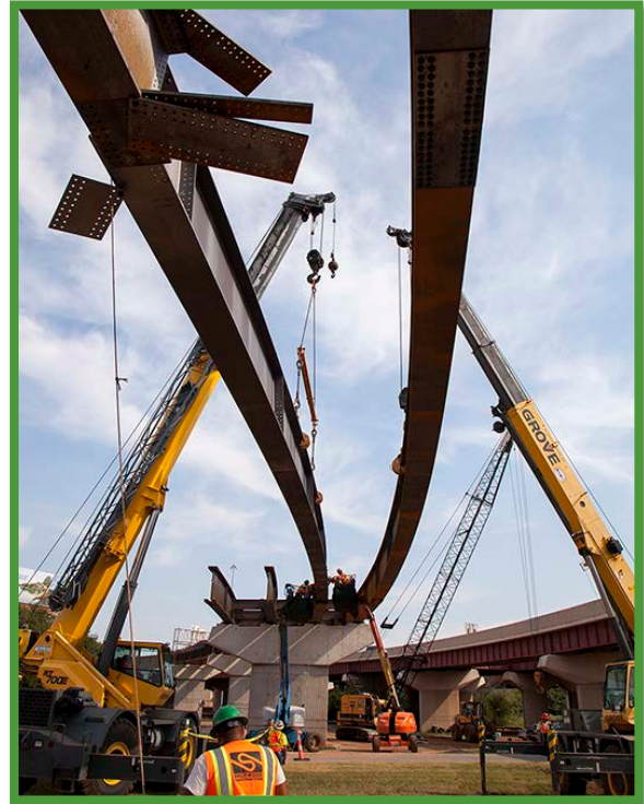
Figure 6: Crews hanging the second beam for the southbound I-235 off ramp to OKC Boulevard for the I-40 Crosstown Relocation in 2015
