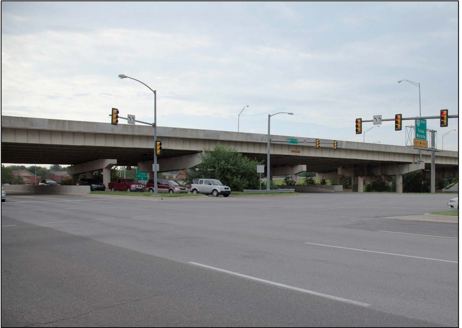
At their Monday, Sept. 8 meeting, members of the Oklahoma Transportation Commission voted to award a more than $3 million contract with potential financial incentives for early completion for a bridge rehabilitation project on the heavily-traveled I-44 Belle Isle bridge in Oklahoma City, pictured here as it crosses over Northwest Expressway.
