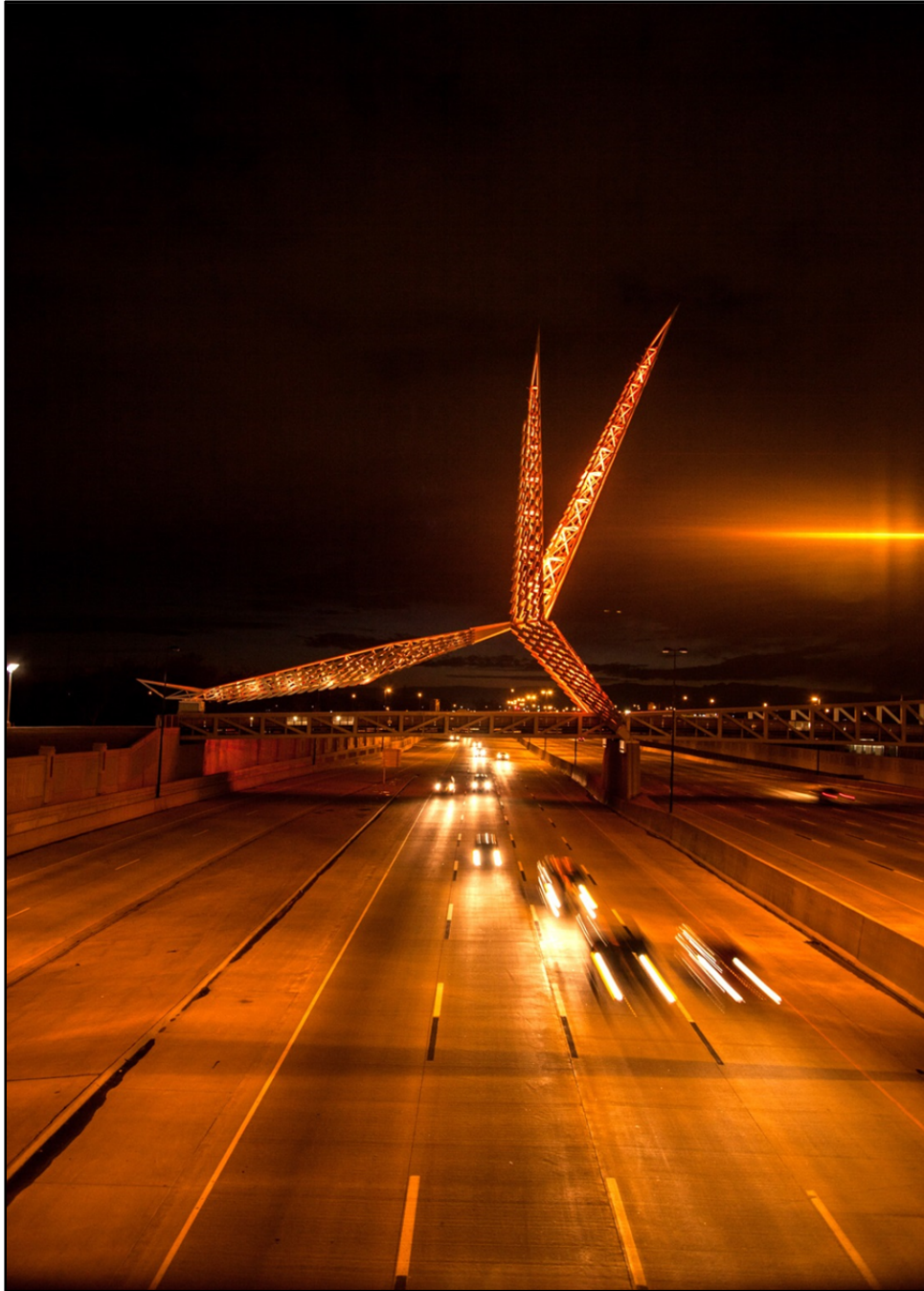
The Skydance Bridge over the I-40 Crosstown in downtown Oklahoma City glowed orange on Monday, April 7 in honor of Work Zone Awareness Week, a national campaign to increase public awareness of the increased number of highway work zones and the crews working in them.
