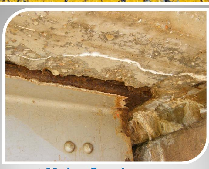
Rusted Steel and Cracked Concrete
