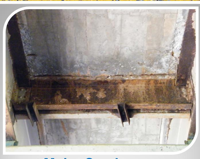
Rusted Steel and Cracked Concrete
