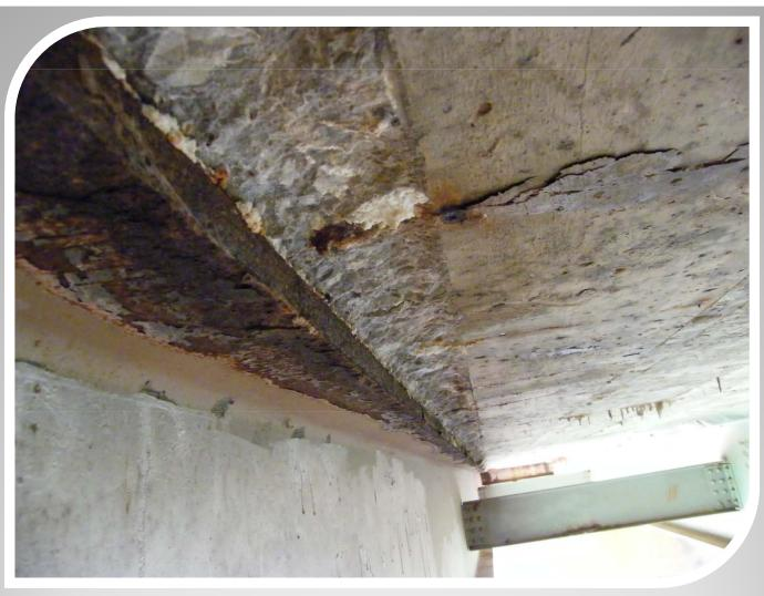
Rusted Steel and Cracking Concrete
