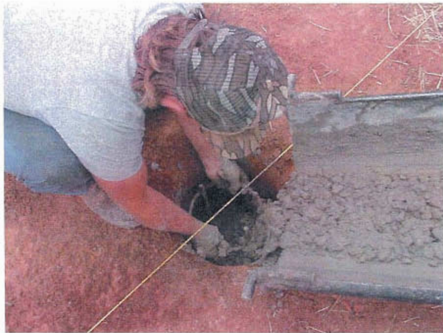
Figure A - 3: Insertion of rebar cage into drilled anchor base hole and concrete placement
