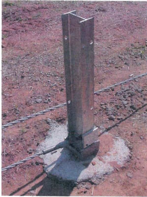
Figure A - 5: Anchor post installed
