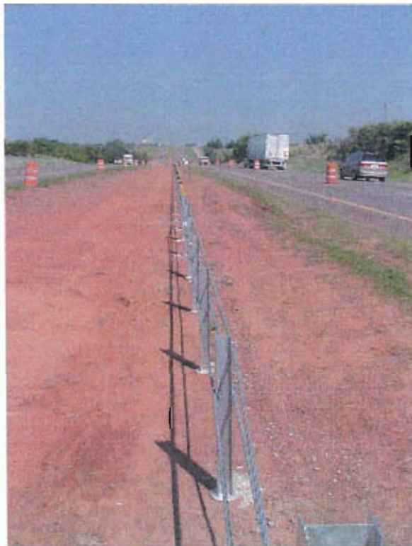
Figure A - 11: Finished cable barrier system.
