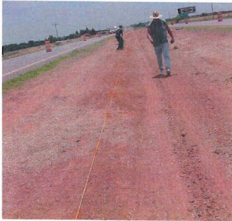
Figure A - 8: Laying out placement of barrier posts.
