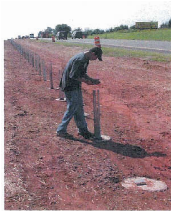
Figure A - 10: Installation of posts and base caps.
