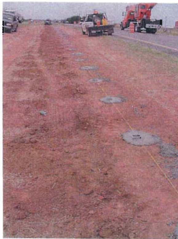
Figure A - 9: Completed barrier post bases.
