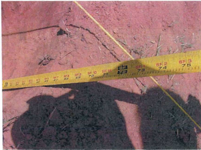
Figure A - 1: Anchor post base hole drilled to depth of 6 feet.
