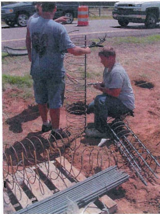
Figure A - 2: Construction of rebar cage for anchor post base.
