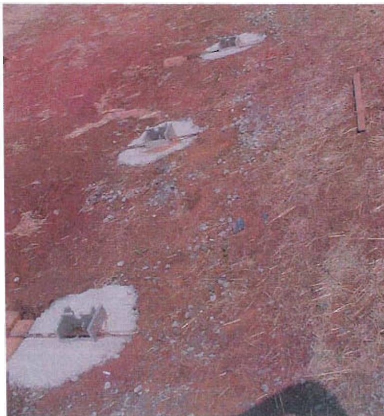
Figure A - 4: Finished anchor post bases.
