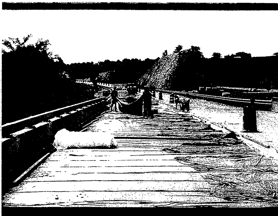
Figure 14. Removing curing blanket on the completed overlay.
