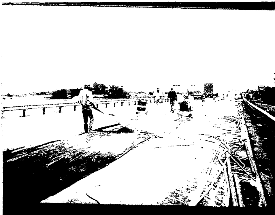
Figure 12. Curing deck with burlap blanket.
