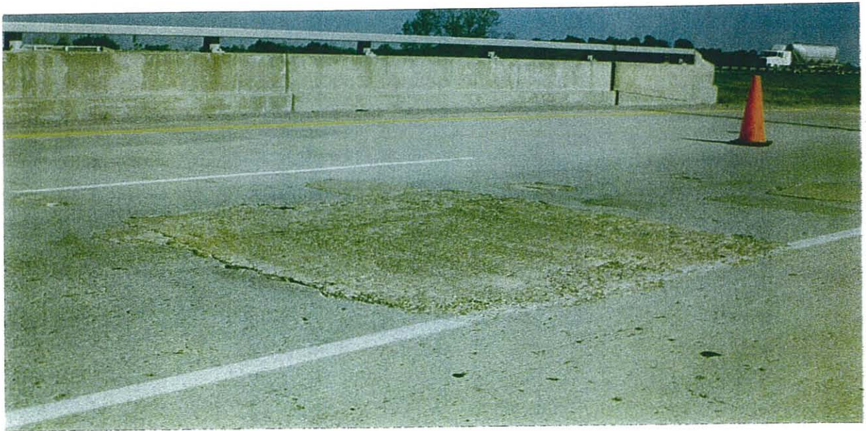
Figure 2. Patching on Existing Bridge Deck, Before Overlay.
