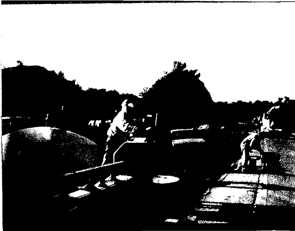
Figure 2. Mixing grout for overlay bond strength.
