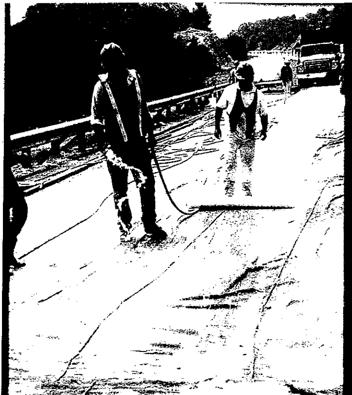
Figure 13. Wetting burlap and covering overlay with plastic for 72 hours.
