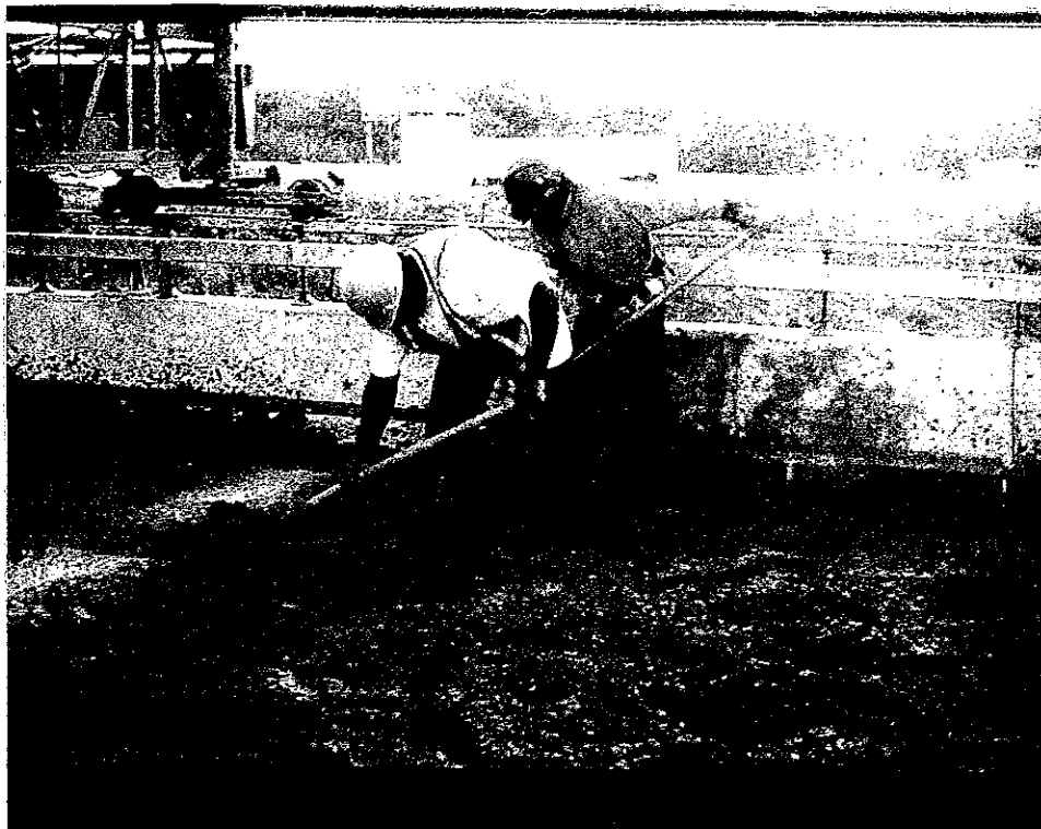
Figure 4. Spreading silica fume concrete by hand.
