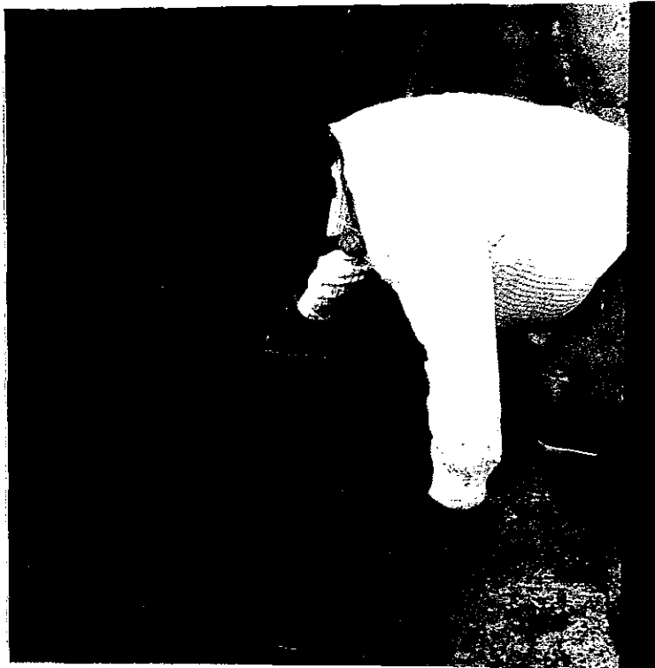
Figure 7. Repairing pits by hand left by the concrete paver.
