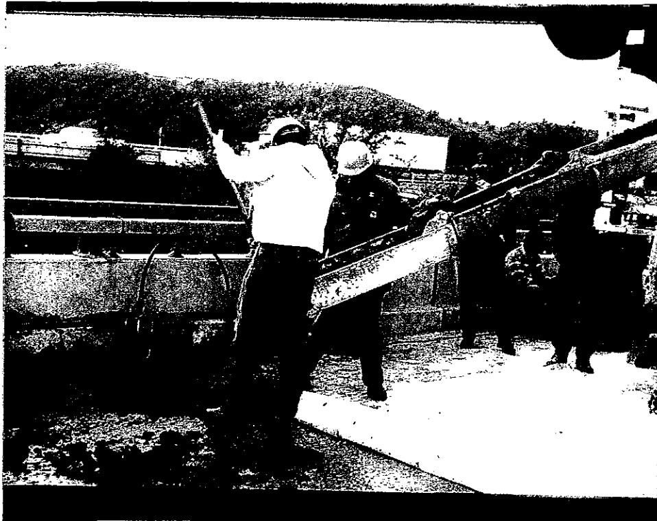
Figure 3. Spreading silica fume concrete for the overlay.
