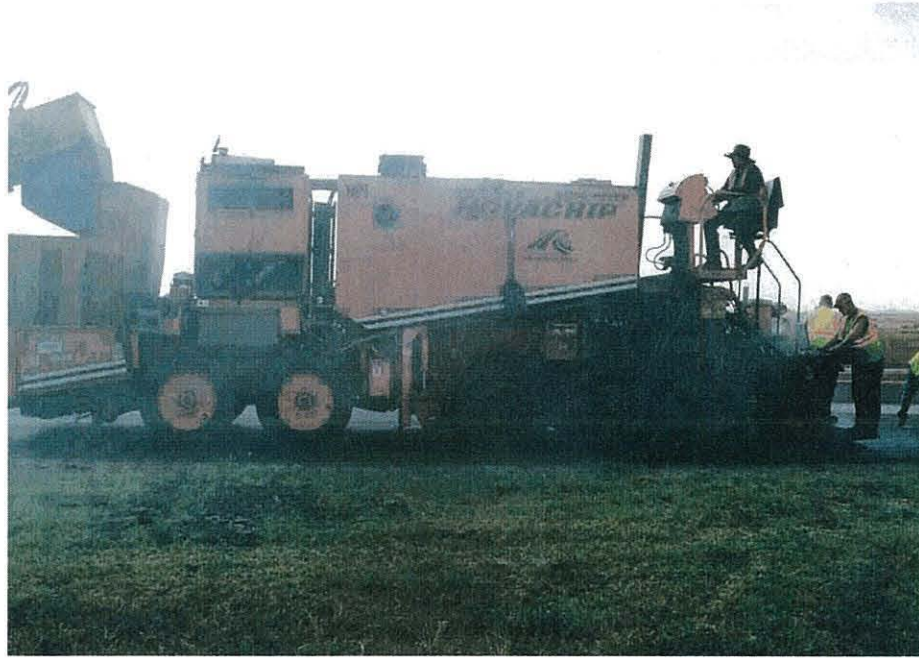
Figure 4. A NovaChip laydown machine.
