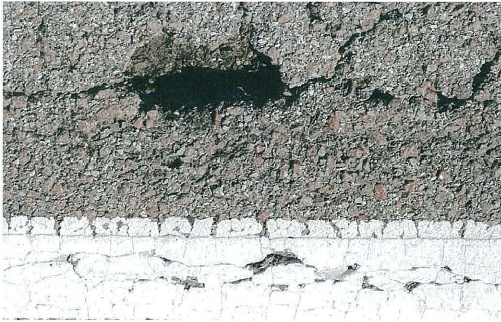
Figure 1 A small pop out and cracking.
