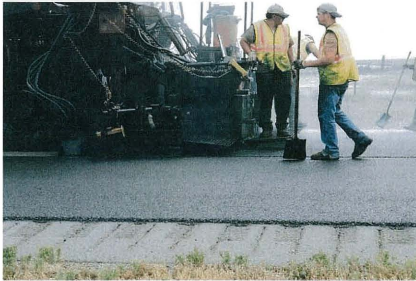
Figure 6. Placing a NovaChip mat.
