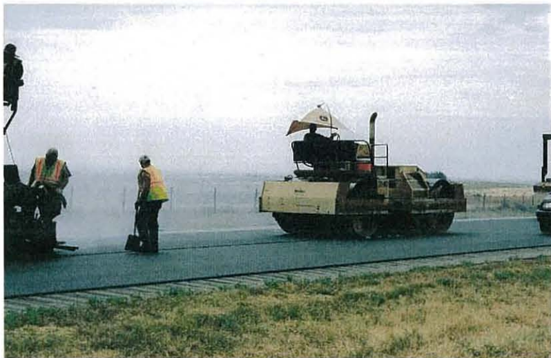
Figure 7. Connell Construction Company rolls Novachip.
