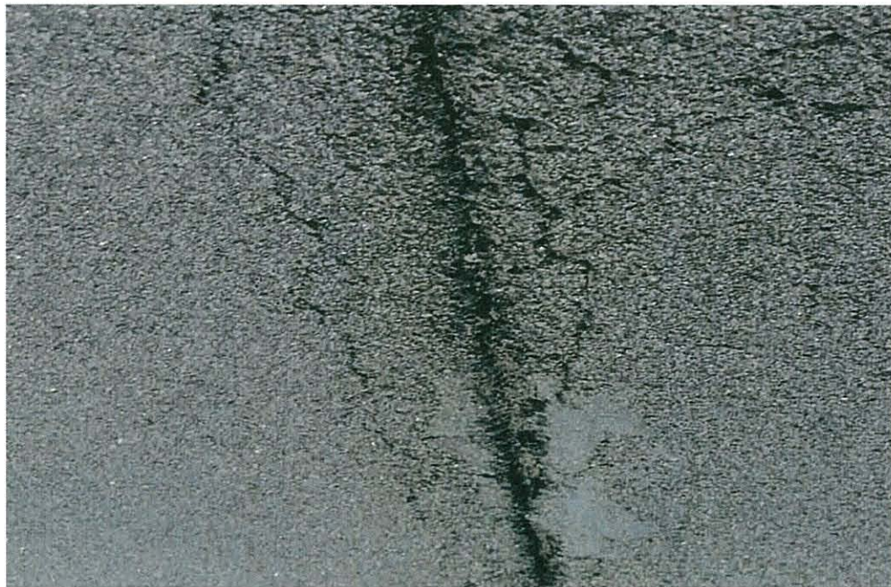
Figure 2. Centerline raveling and cracking.
