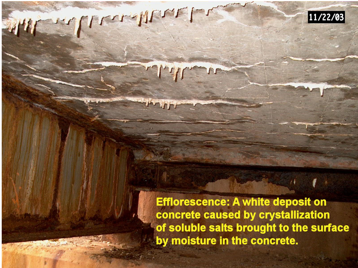
Figure 520:1. Photo. Efflorescence
