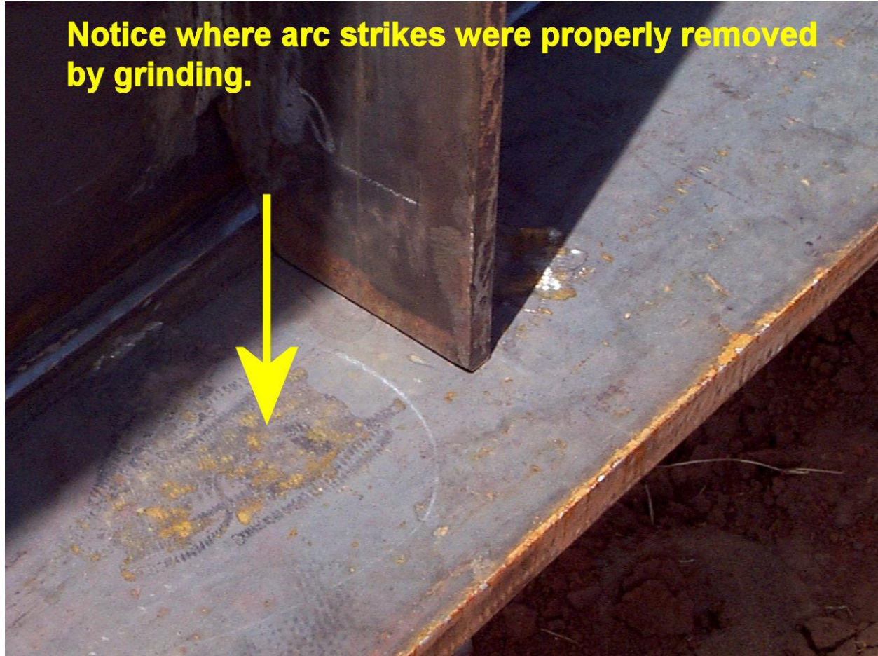
Figure 506:6. Photo. Proper Removal of Arc Strikes by Grinding
