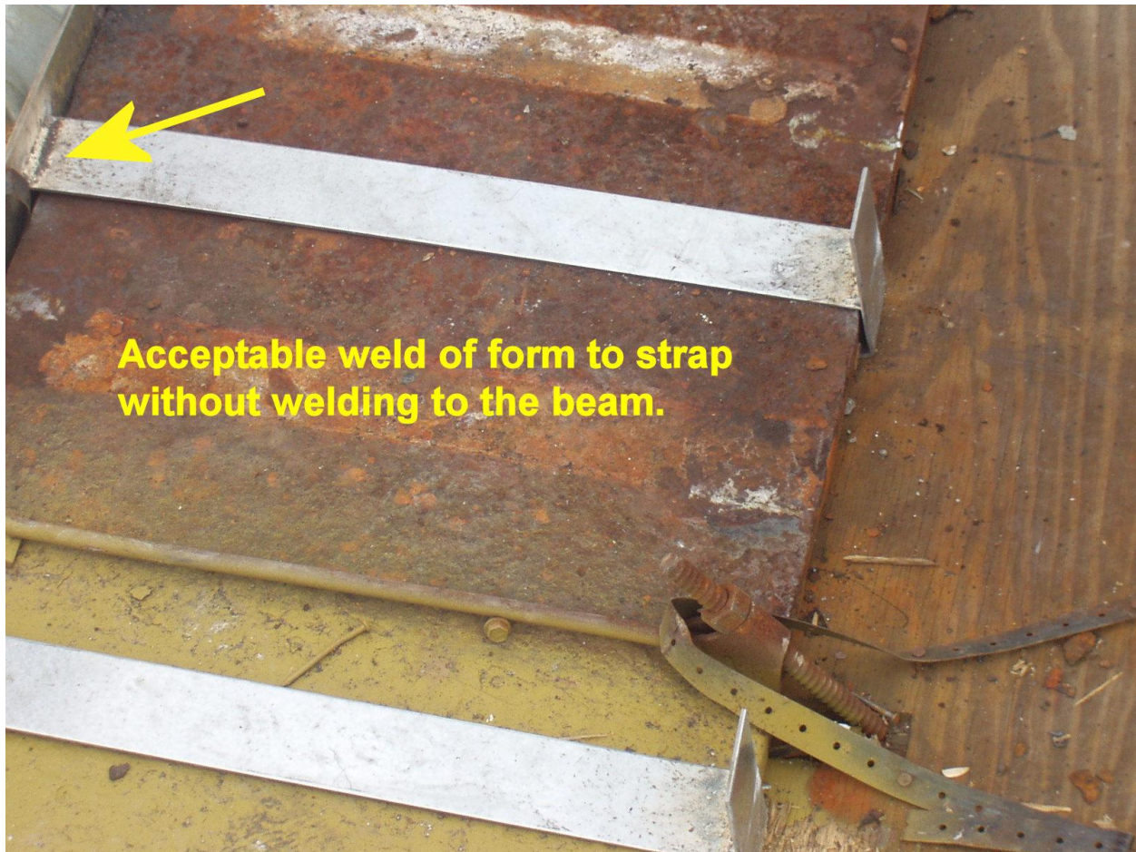
Figure 502:6. Photo. Acceptable Weld of Stay-in-Place Forms
