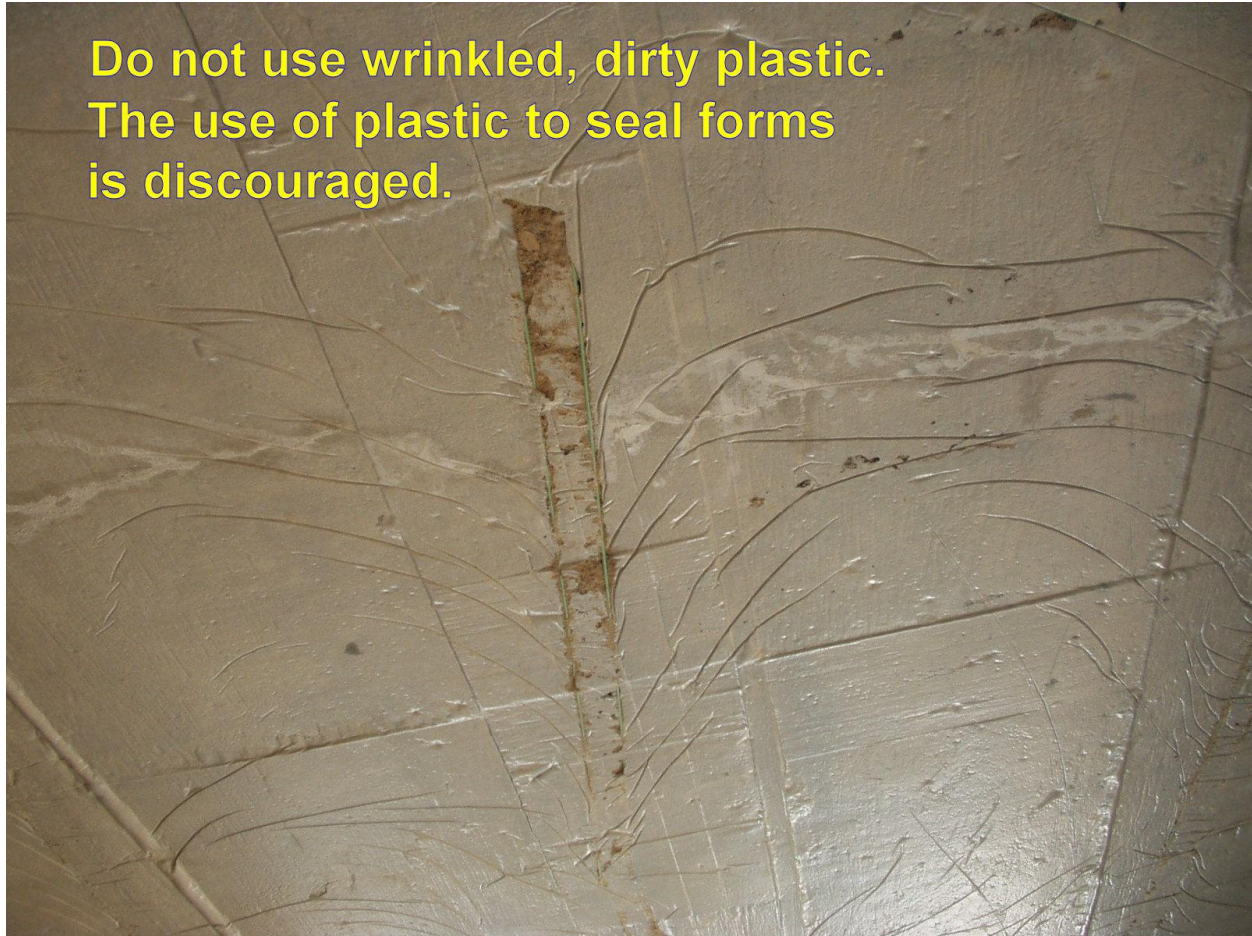
Figure 504:1. Photo. Sealing Forms with Plastic
