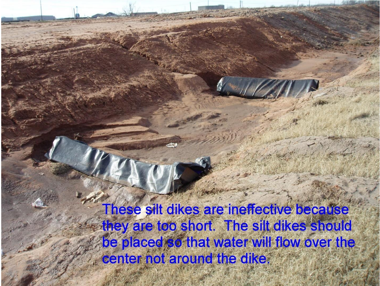
Figure 221:4. Photo. Ineffective Silt Dikes
